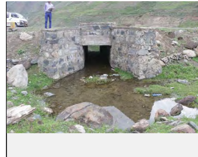
View of Box Culvert at the toe of slope
