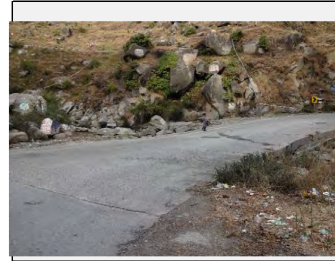
Road condition: The causeway is installed crossing the stream.
