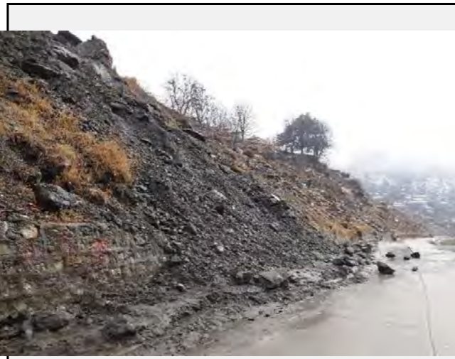
Existing countermeasures / anomalies: The slope failure is causing rocks on the road.
