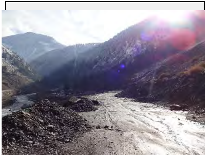
Existing countermeasures: Temporary access road used for the long-sized truck which cannot pass the road alignment on the bypass road.
