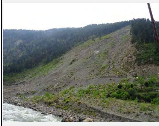
Overall view of the slope from the opposite site of the river. Talus deposited on whole surface of the slope failure area.
