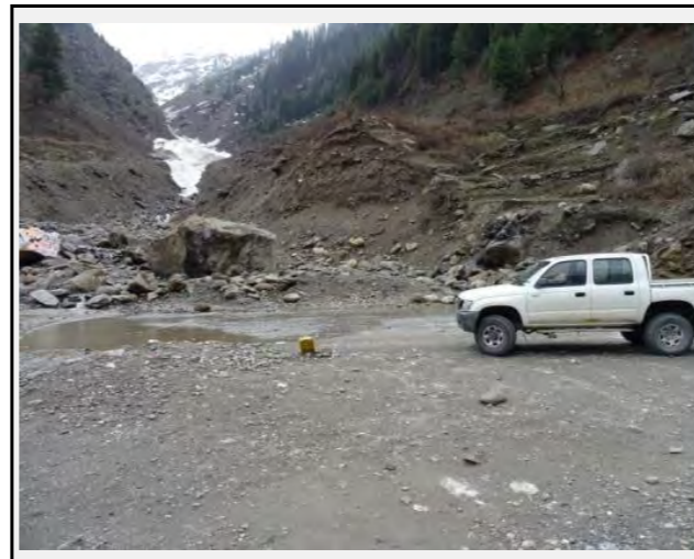
Big sized boulders (5m*8m*3m) can be seen on the stream bed. The Sides of the stream are completely bare and highly erodable
