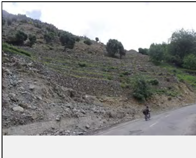
The Check dams has been built along the debris flow
