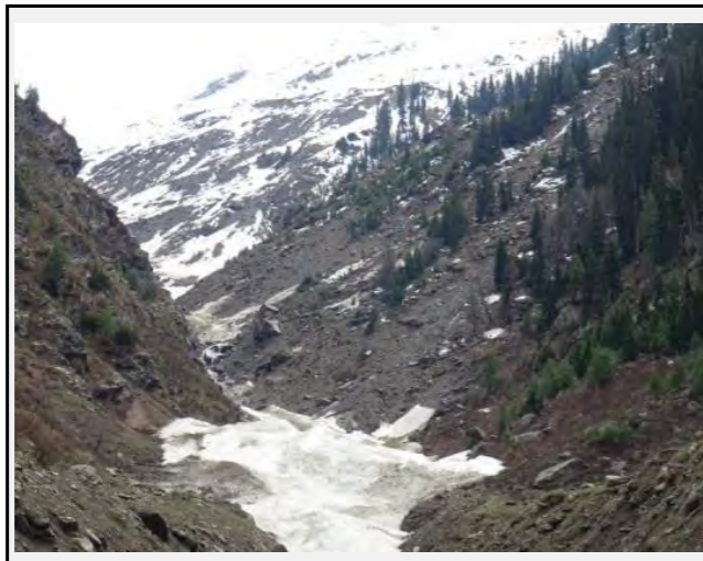
There is a big collapsed slope in the water catchment area
