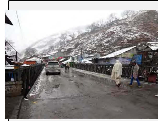
Road condition: No anomalies was confirmed on the road ( bailey bridge)
