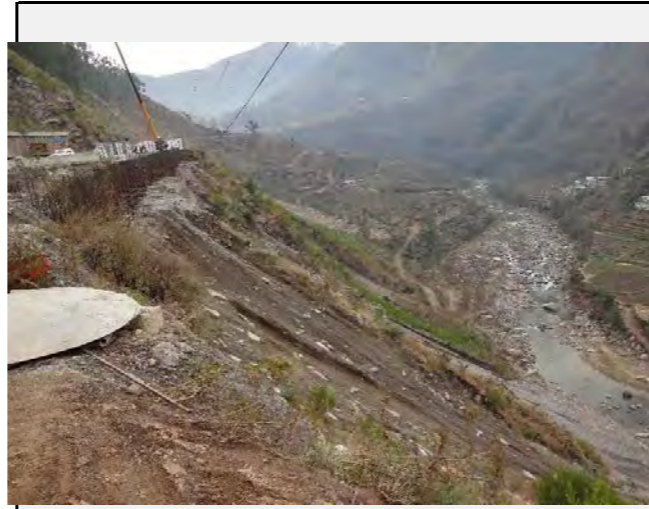
Valley side: Talus deposit can be observed on the valley side of the slope
