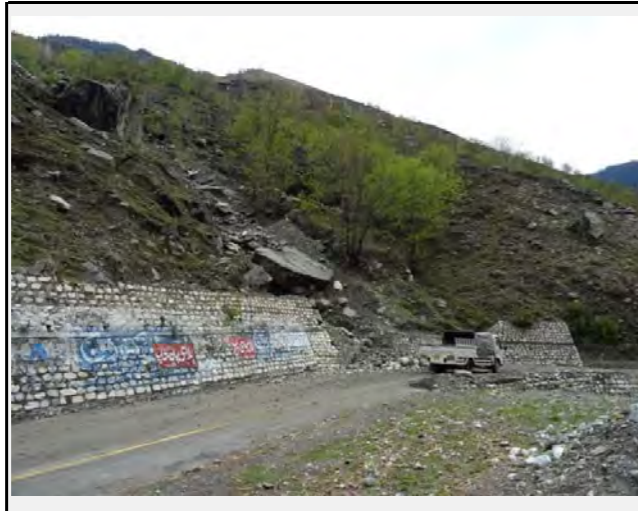
Mountain side: Big boulders (2~5m) can be observed at the exit of the stream on the mountain side.
