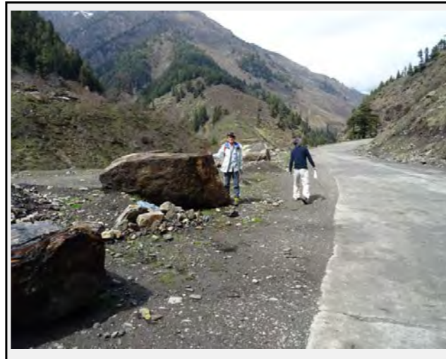
The biggest fallen rock identified (2m*1m*1m) has been pushed to the road side
