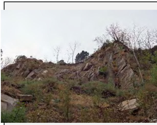
Existing anomalies: Unstable rocks can be observed at the top part of the slope. The stacks are also mostly vertical.
