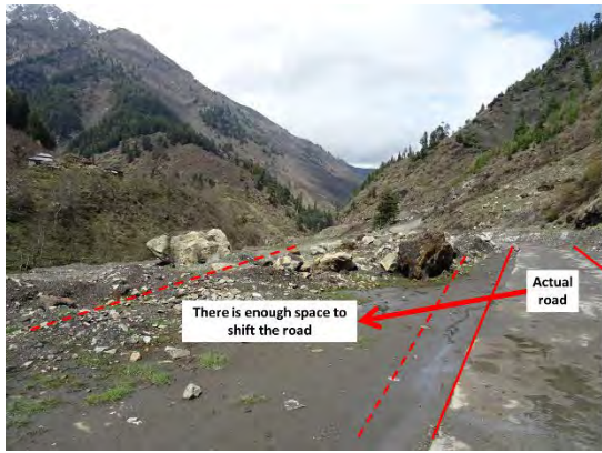
Figure 4.66 Road can be shifted toward the Valley Side because there is enough flat space (Example in N15_8). It should be Noted that shifting the road does not mean the disaster can be avoided
