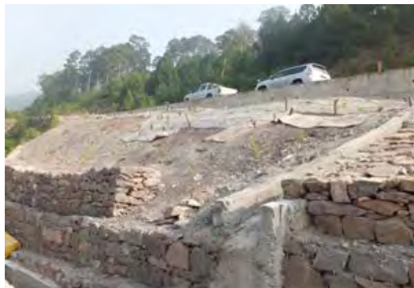
Figure 4.42 Masonry on the Valley side of N75 Source: JICA Survey Team
