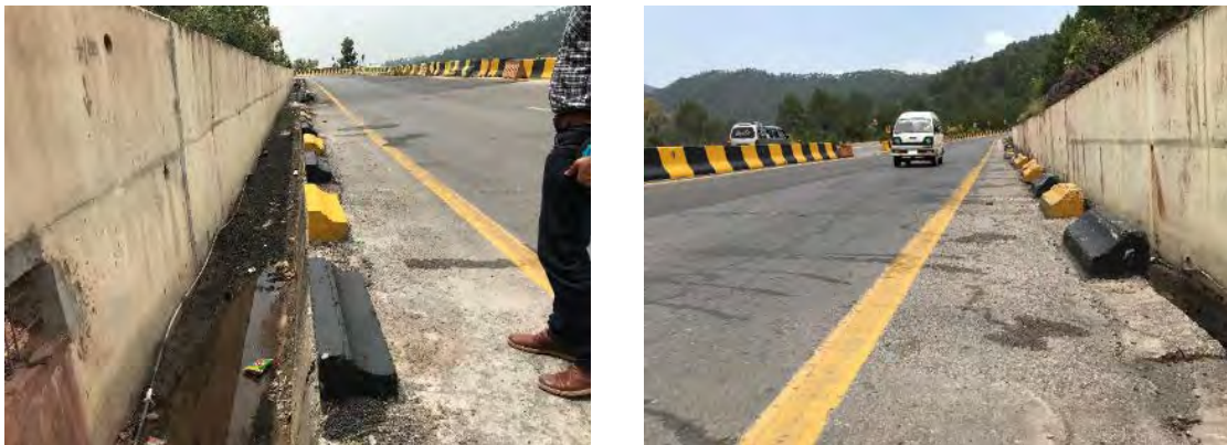
Figure 4.50 Puddle in the Ditch (Left), Situation of the Surface Drainage (Right) at N75_2
