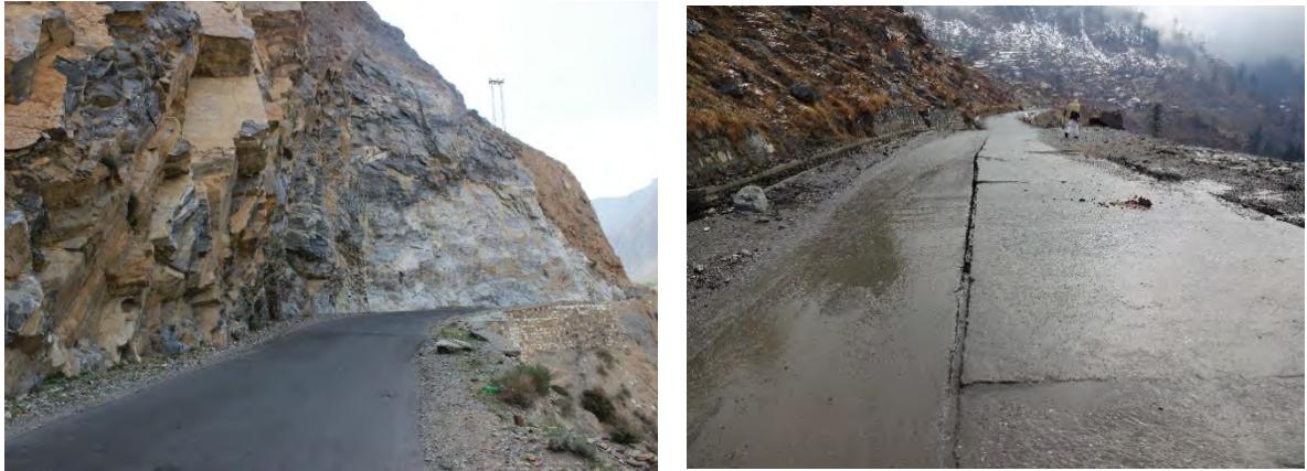
Figure 4.41 Inadequate Cut Slope Angle (Left) and Lack of Bearing Capacity of Embankment (Right)
