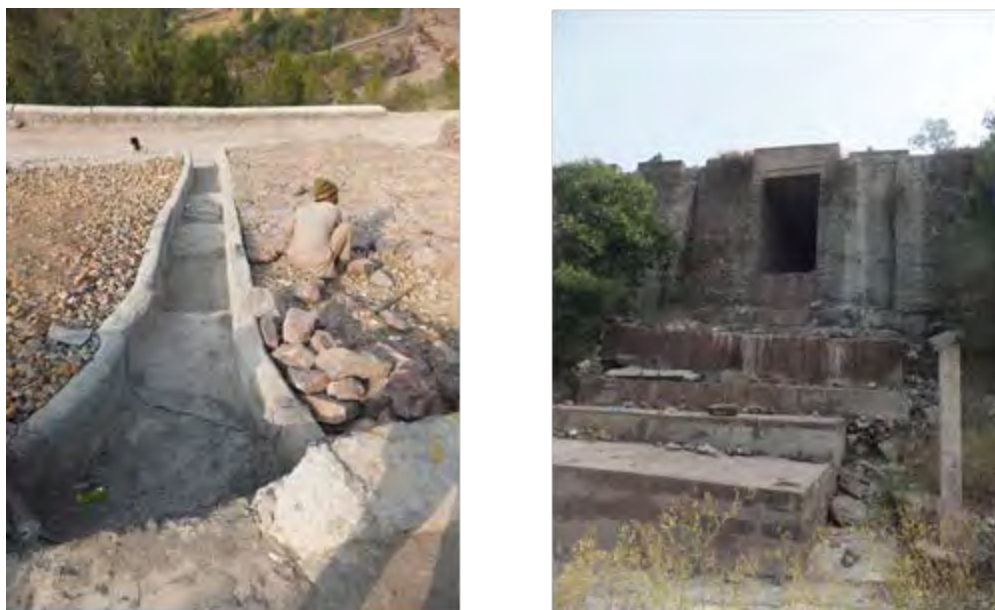
Figure 4.43 Surface Drainage on the Valley side (Left) and Box Culvert Crossing the Road (Right): Both functions are to Reduce Flow Speed Source: JICA Survey Team
