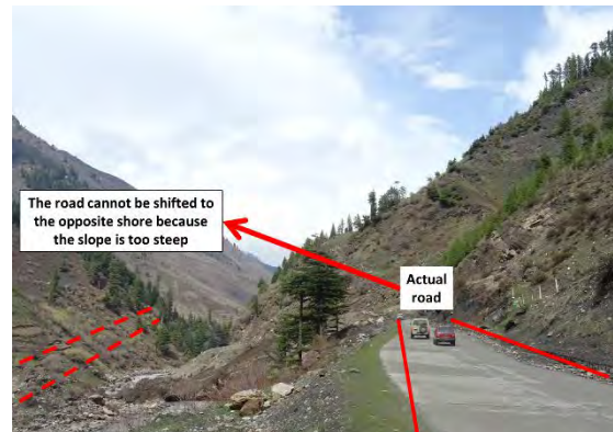
Figure 4.69 Similar Road cannot be Constructed in the Opposite Shore because the Slope is too Steep. (Detouring is not Possible by Construction of a Bridge) (Example in N15_8)
