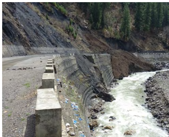
Figure 4.36 Vertical Slope of (N15_8) and Collapsed Retaining Wall (N15_9)
