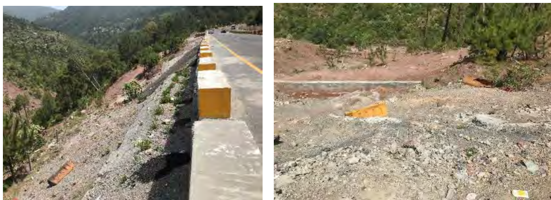
Figure 4.48 Inadequate Construction of Embankment on the Valley side Slope at N75
