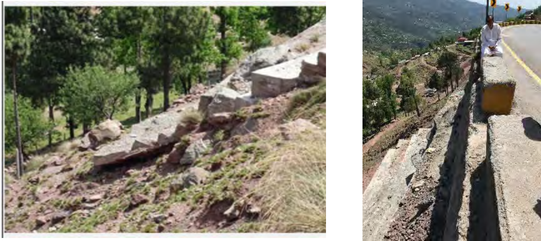
Figure 4.49 Inadequate Construction of Retaining Wall on the Valley side Slope at N75_5
