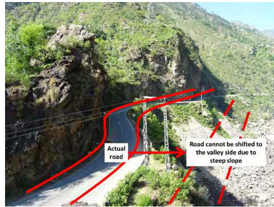
Figure 4.67 Road cannot be shifted toward the Valley Side because there is not enough flat space (Example in N35_8)
