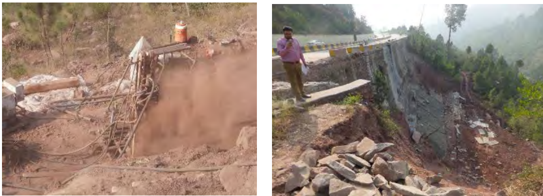
Figure 4.45 Insertion of Micropile (Left) and Failure of embankment in the valley side (Left)
