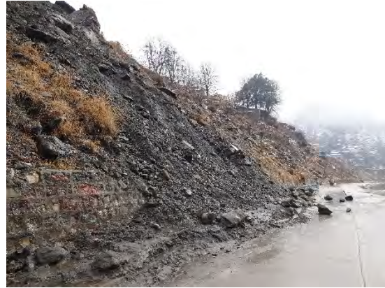
Figure 4.34 Slope Failure Affecting Road Traffic at N15 Source: JICA Survey Team
