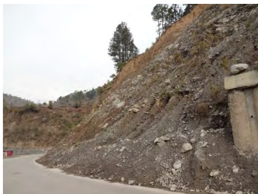
Surface collapse at N35_1
