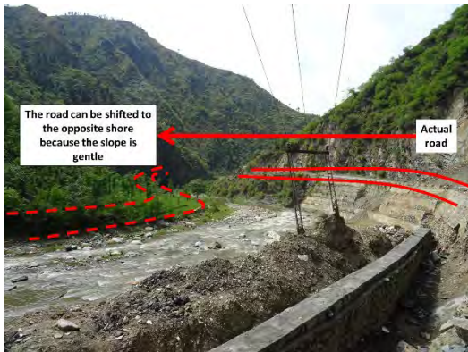
Figure 4.68 Similar Road can be Constructed in the Opposite Shore (Detouring is Possible by Construction of a Bridge) (Example in N35_3)
