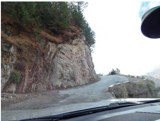
Figure 4.35 Example of Inadequate Angle of Cut Slope and Road Embankment
