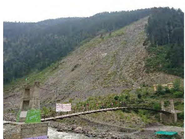
Photograph 6: Slope failure (N-15)
