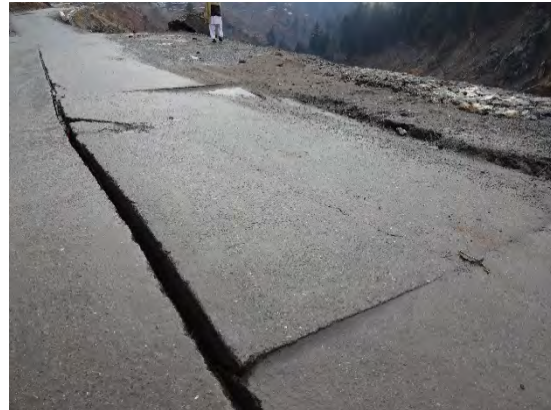
Figure 4.35 Example of Inadequate Angle of Cut Slope and Road Embankment
