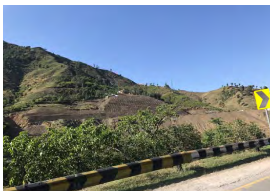
Figure 4.52 Situation of Slope Stabilization along N35 by Chinese Company (Between Havelian and Abbotabad) Source: JICA Survey Team
