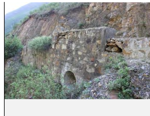
View of Drainage pipe and damaged retaining wall
