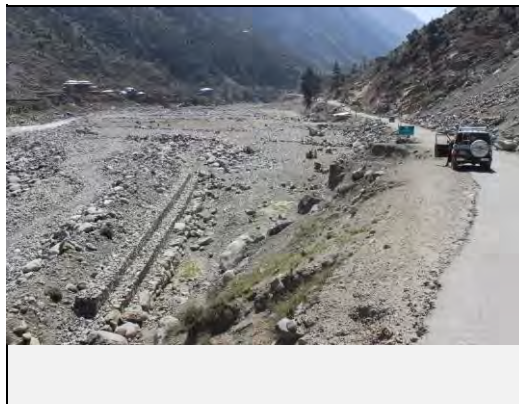
View of slope failure on Valley side and a river diversion structure built at the toe of the slope failure
