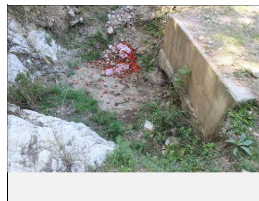
Existing countermeasures / anomalies: View of culvert inlet at the toe of slope failure
