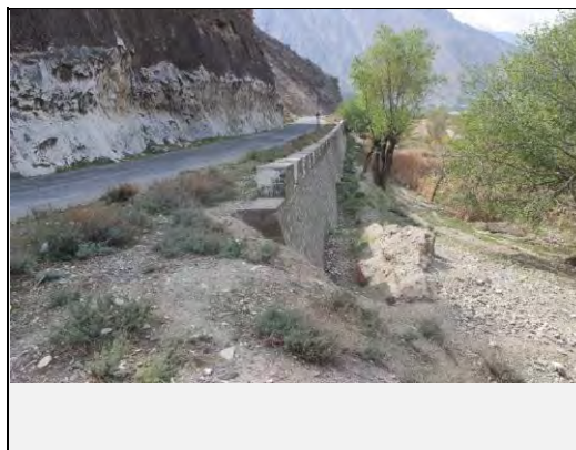
View of Slope Failure on Valley side:
