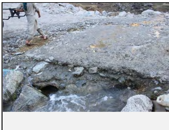
The damage on road has been observed with inlet of pipes for debris flow
