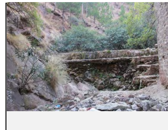
Existing countermeasures / anomalies: Benches has been made on the upstream which has been partially destroyed
