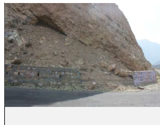
View of unconsolidated material with damaged retaining wall.
