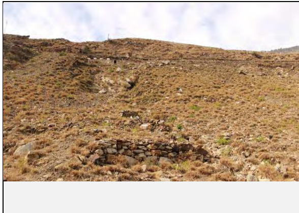
Full view of the landslide
