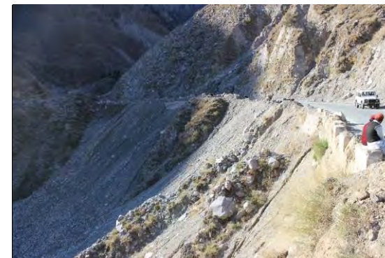
View of fallen blocks
