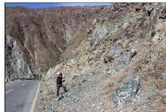
View of Large blocks fallen and talus deposit at the toe of Sloape Failure
