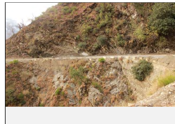
Existing countermeasures / anomalies: Retaining wall has been constructed at the toe of the slope failure
