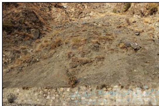
Full view of the landslide
