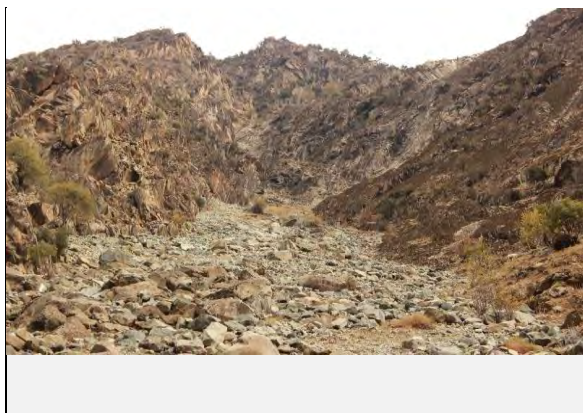
Full view of the landslide
