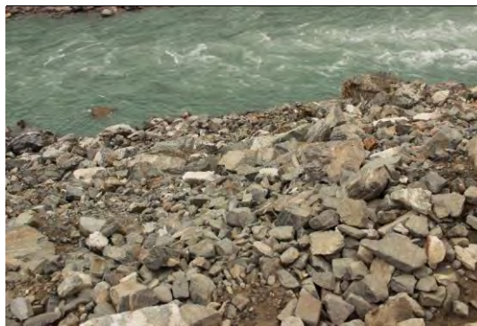
View of landslide on Valley side:
