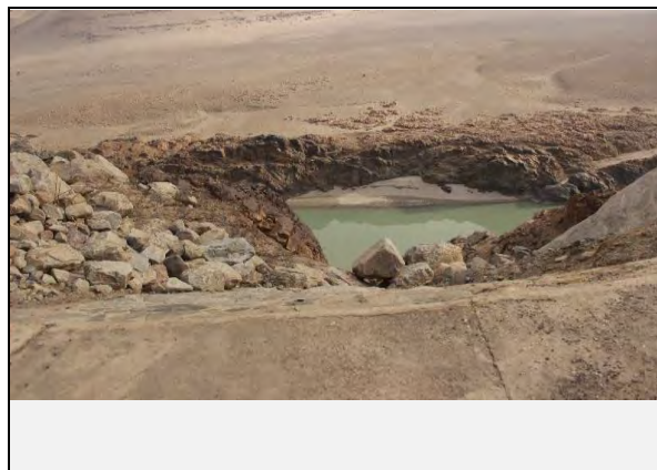
Valley side view of the debris flow
