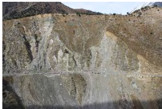
Full view of the landslide
