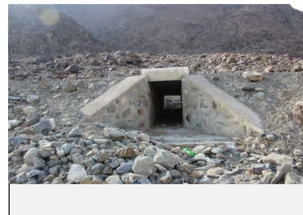
Existing countermeasures / anomalies: Culvert outlet view
