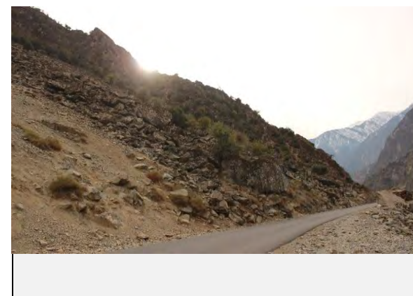
View of fallen blocks
