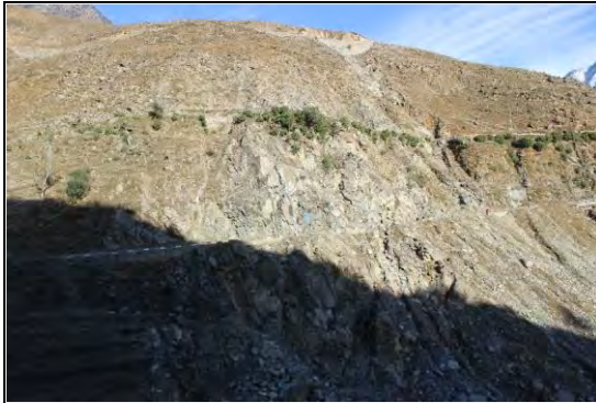
Full view of the landslide
