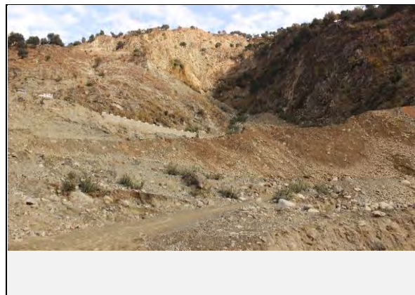
Full view of the landslide
