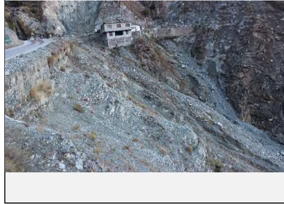
View of landslide on Valley side:
