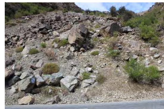
View of fallen blocks
