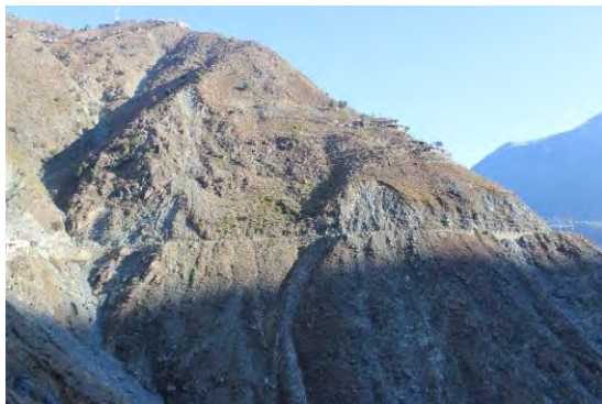
Full view of the landslide
