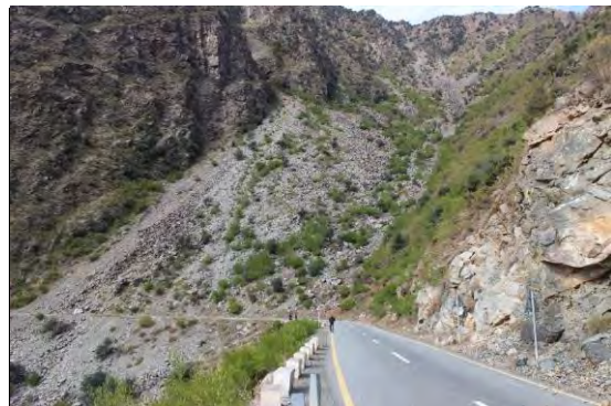
Full view of the landslide
