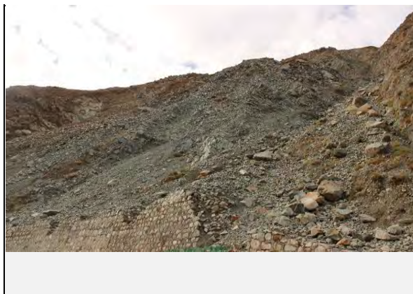
Full view of the landslide
