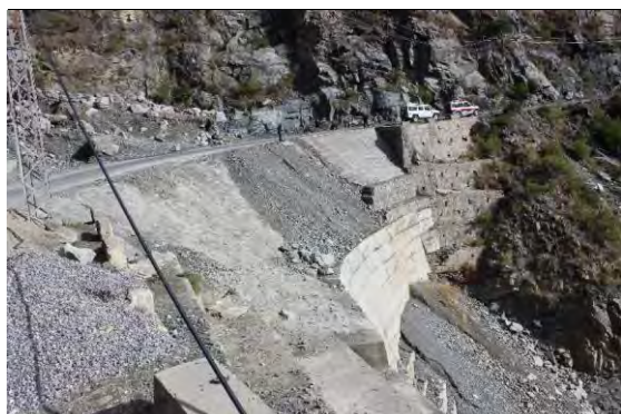
Existing countermeasures / anomalies: Sloped Retaining wall has been constructed for Debris material
