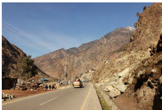
View of landslide on Valley side:
