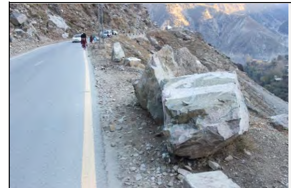
View of fallen blocks on road
