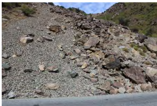
Existing countermeasures / anomalies: No counter measures
