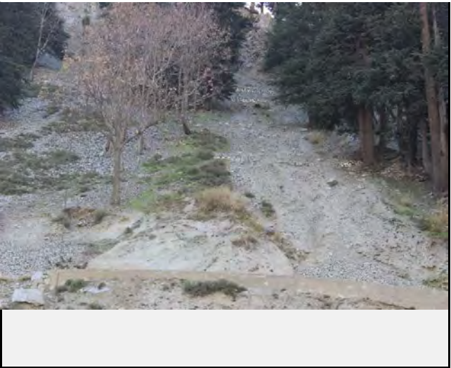
Existing countermeasures / anomalies: View of check dams as counter measure
