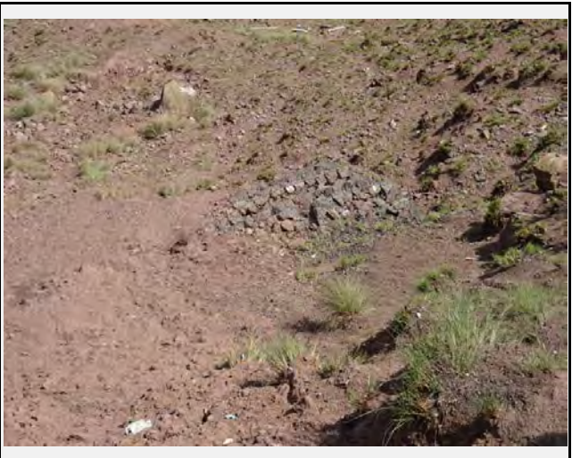
Slope failures have collapsed and damaged gabion walls constructed in the valley side as retaining walls for the embankment
