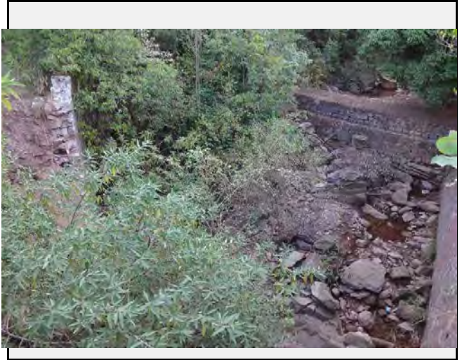
Existing countermeasures / anomalies: Damage on the retaining wall on the north side (undercut slope) on the mountain side.
