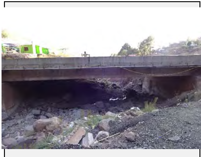
Existing countermeasures : The height underneath the bridge seems enough to clear the debris to the valley side.
