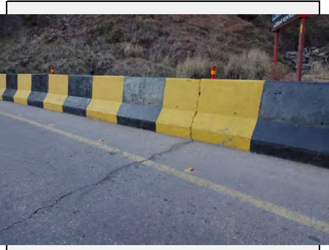
Road condition: Some cracks was observed at the joints of the bridge.
