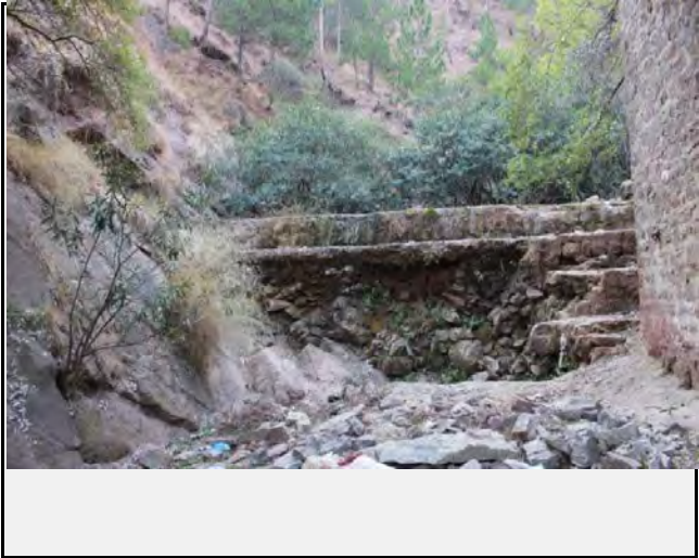
Existing countermeasures / anomalies: Benches has been made on the upstream which are been partially destroyed
