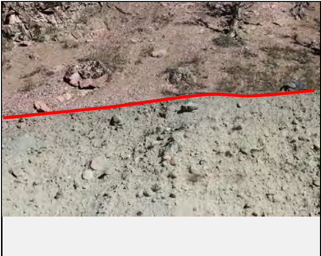
The existing road has been damaged. Red line shows the old road displaced by the debris flow.
