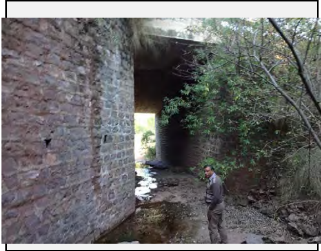
Existing countermeasures / anomalies: The box culvert are clear from any debris.
