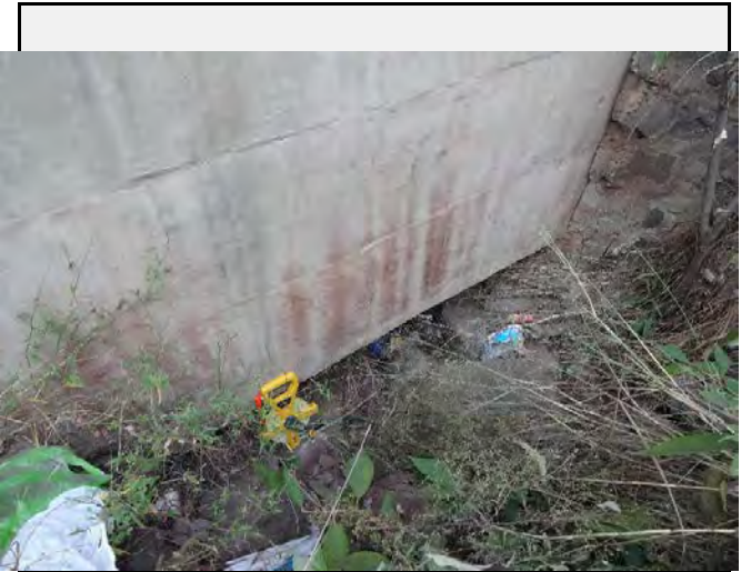
Existing countermeasures: The culvert is filled with debris and rocks which may block the waterway from the mountain area, resulting the flooding of the road.
