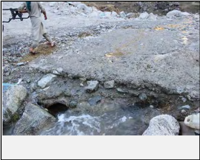
The damage on road has been observed with inlet of pipes for debris flow
