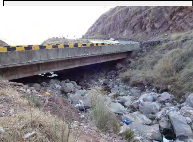
Existing countermeasures / anomalies: Dumping of the garbages around the bridge reduce the capacity to drain the debris to the valley side.
