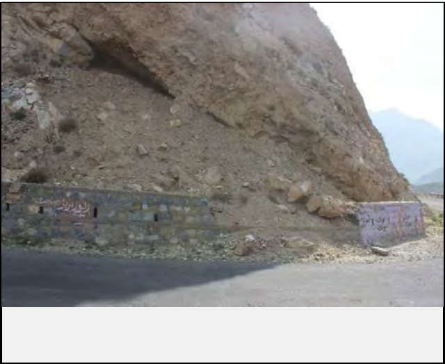
View of unconsolidated material with damaged retaining wall.
