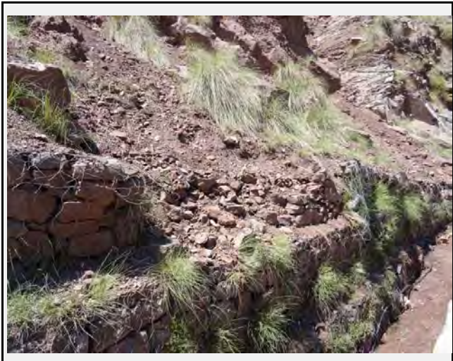
The gabion wall is damaged in many spots due to past rock falls and is thought not to operate properly as a countermeasure
