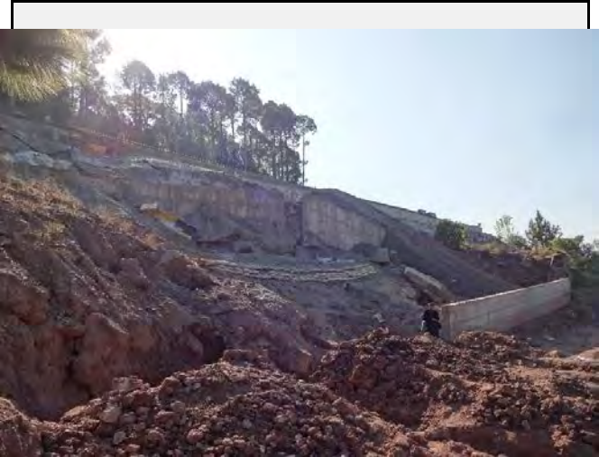
Existing countermeasures / anomalies: Retaining walls are constructed at the valley side of the road (ongoing construction).
