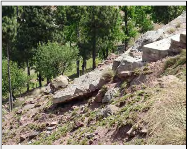
The retaining wall in the valley side is being damaged because the soil on which it is constructed is being washed away.
