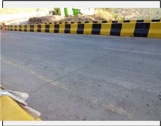
Road condition: Small cracks was confirmed at the joint section of the road and bridge.
