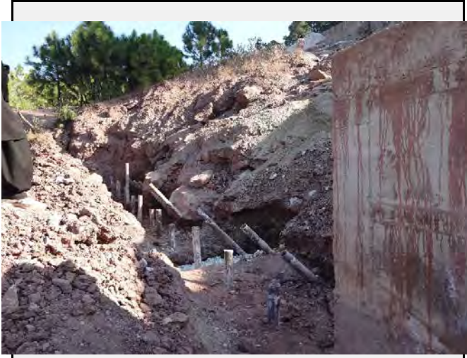
Existing countermeasures / anomalies: Micro piles are installed at the foundation of the lowest retaining wall (ongoing construction).
