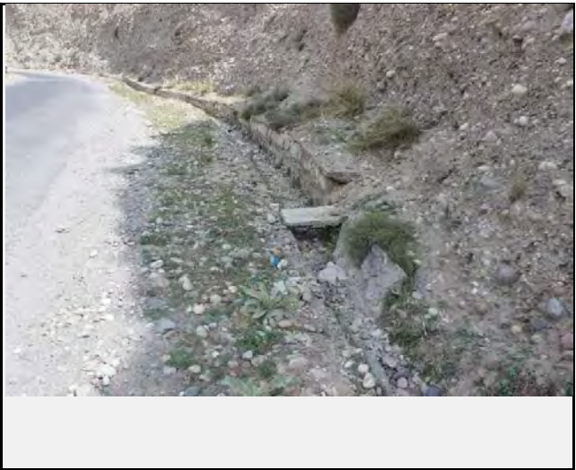
Existing countermeasures / anomalies: View of channel at the toe of Slope Failure
