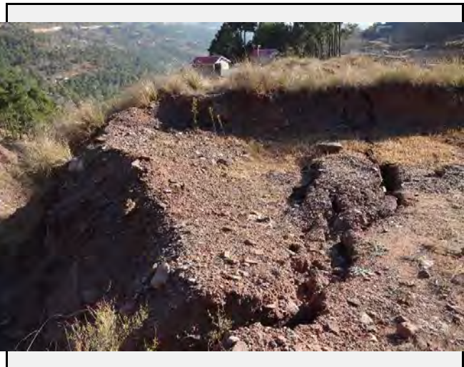
Existing anomalies: Cracks was confirmed on the bank of the valley side. It may collapse in near future due to the erosion.
