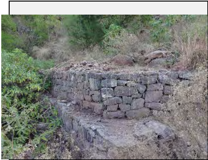
Existing countermeasures: Gabion works are undertaken at the toe of the mountain side. However, the debris is deposited on the top of the gabion and may outflow the gabion works in the future.
