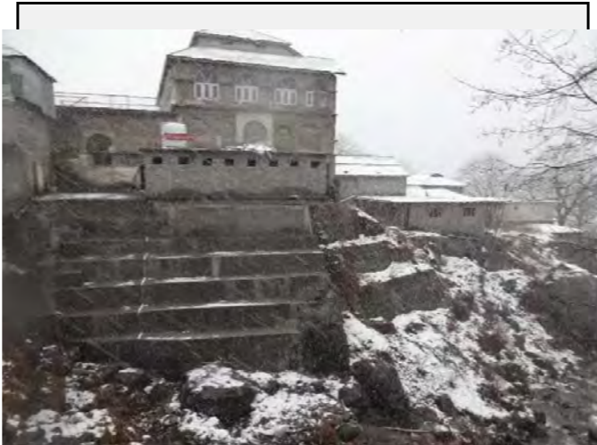
Existing countermeasures: Retaining wall is constructed on the both side of the bridge to protect the bank erosion.
