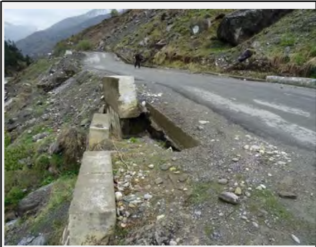
Road condition: Two area of the road subsidence was confirmed. There might be a cavity underneath the road.
