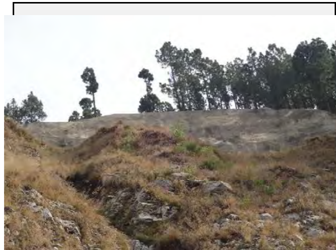
Existing countermeasures : Shotcrete was undertaken by FWO on the head of the slope to minimize the surface erosion.
