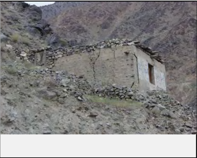
Existing countermeasures / anomalies: No Counter Measure. House has been damaged along the Debris Flow
