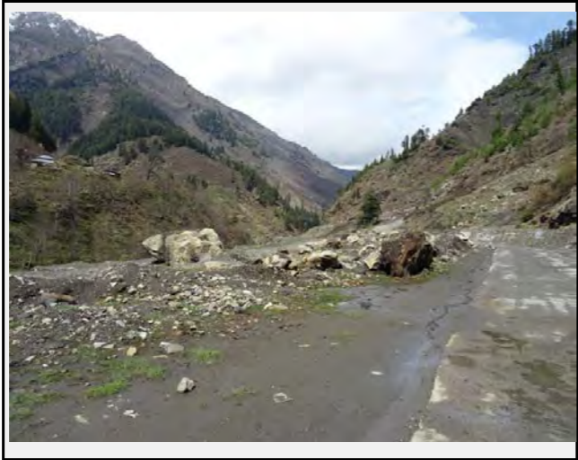
There is evidence of rock falls in the past that have been pushed to the valley side to clear the road
