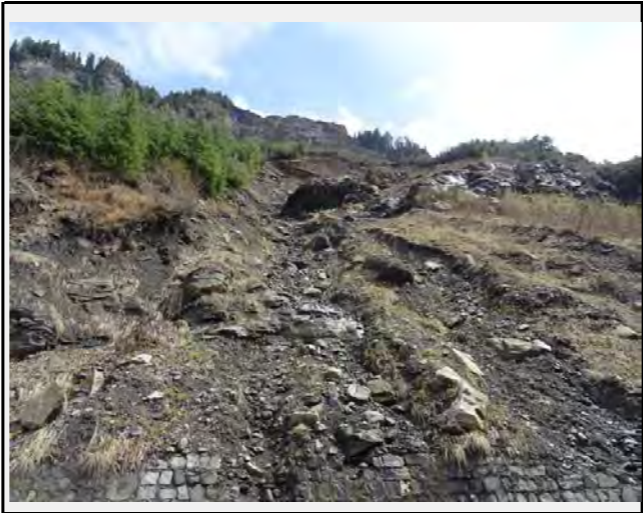
Fallen rocks that have not reached the road but may collapse and fall again can be identified throughout the slope
