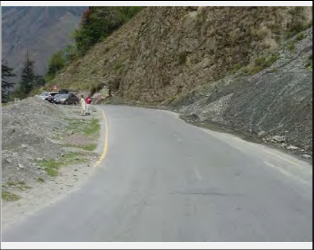
Road condition: road ditch is covered by debris
