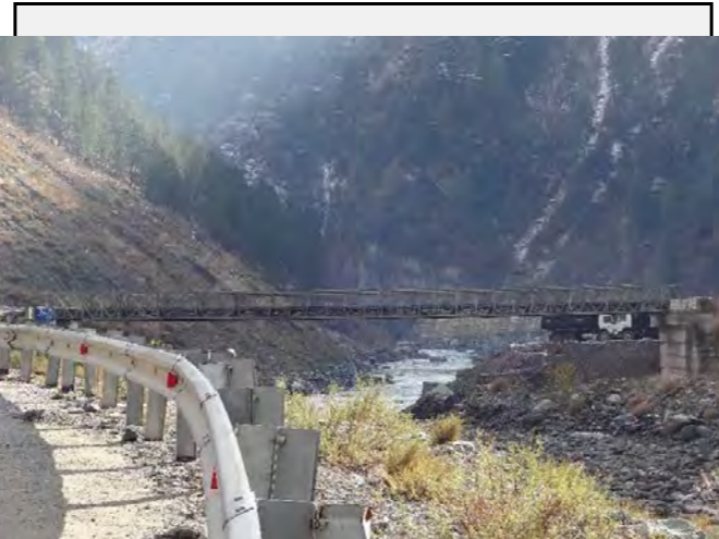
Existing countermeasures: Bailey bridge is used as temporary on the bypass road.
