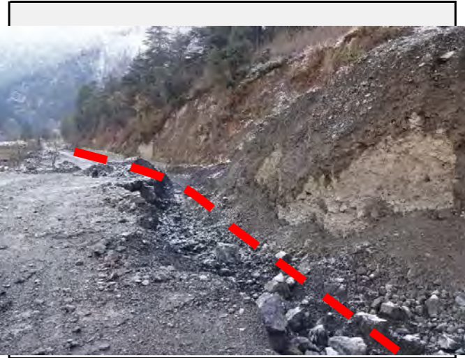
Road condition: Existing road is still buried 5m under the talus deposits.
