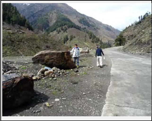
The biggest fallen rock identified (2m*1m*1m) has been pushed to the road side
