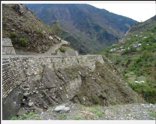
Possible countermeasures: a bridge can be constructed in the valley side of the road avoiding the debris flow stream.
