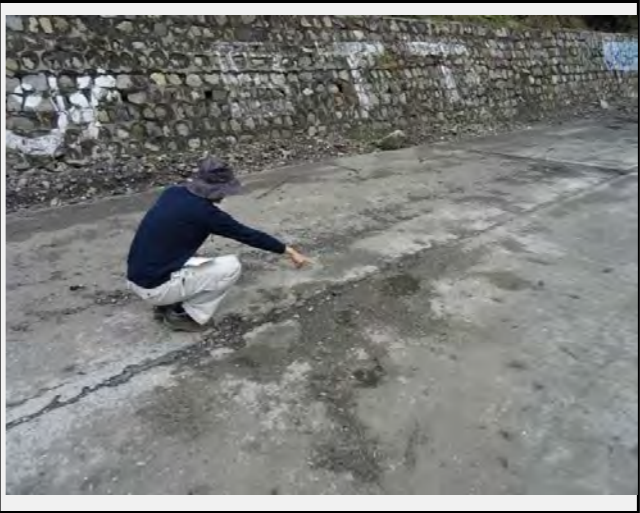
The rock falls cause damage on the road bed forming pot holes
