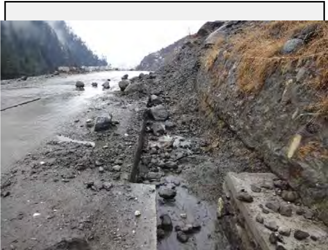
Existing countermeasures / anomalies: Some part of the water canal are filled with the debris.
