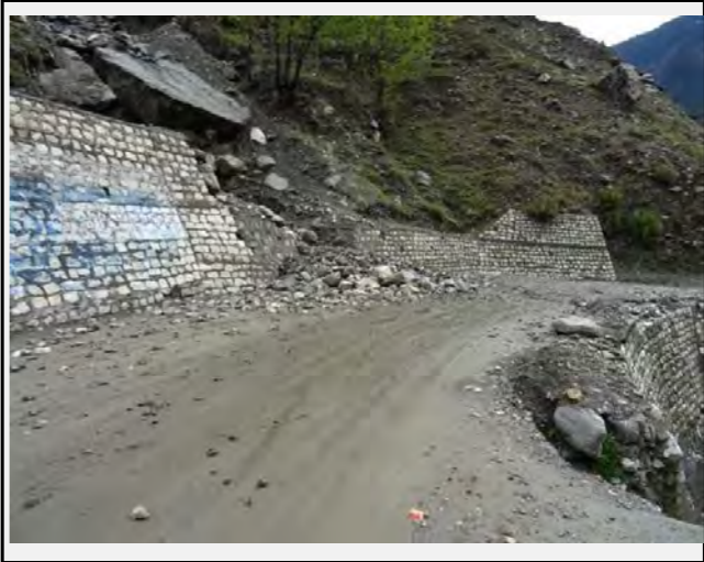
Road condition: there is mud and debris on the road and the road surface is damaged considerably
