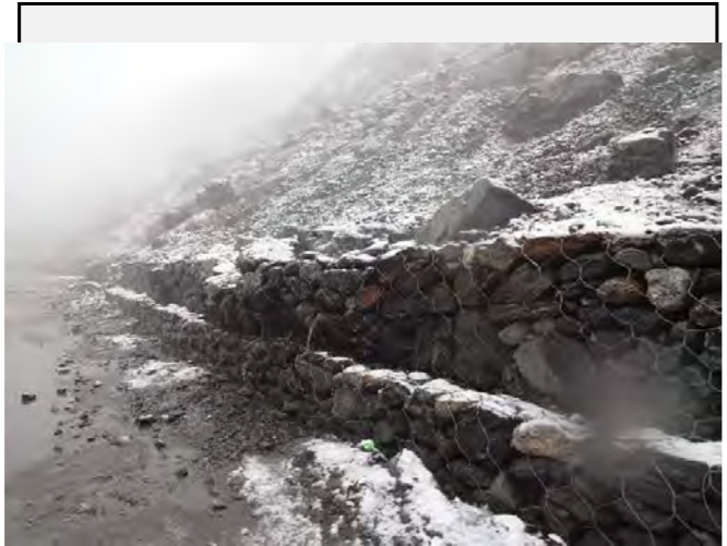
Existing countermeasures / anomalies: Several damages on the gabions was confirmed due to overload of the deposit.
