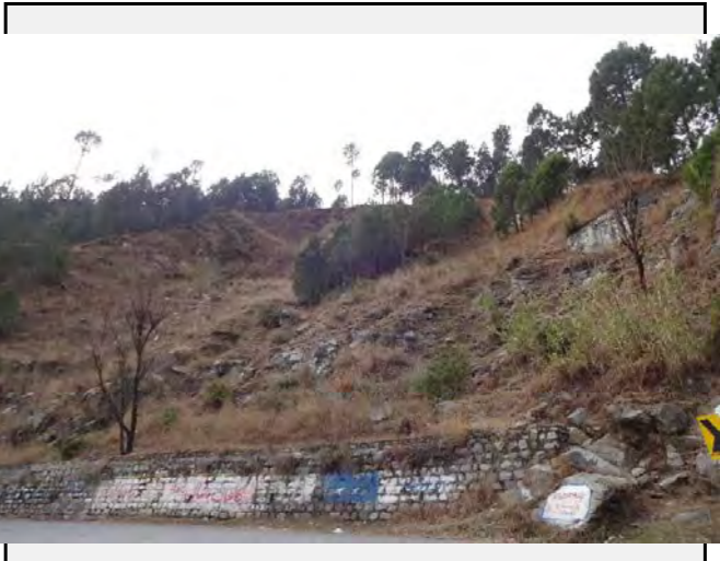
Others: Trace of the slope failure at the side of the stream. Retaining wall is constructed at the toe of the slope. However, the slope is covered with vegetation and seems stable.
