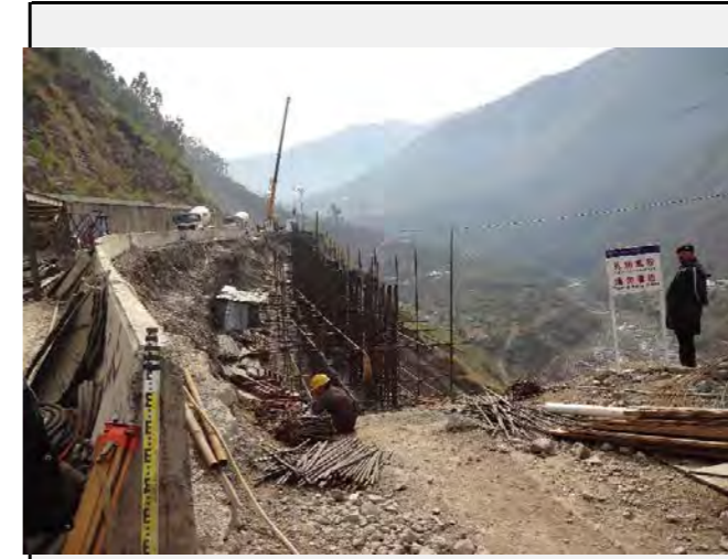
Road condition: Construction on shifting the road alignment to the valley side is being carried out by CPEC.
