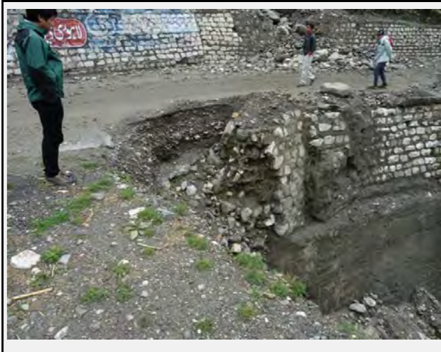
Existing countermeasures / anomalies: small damage (2m) of the retaining wall on the shoulder of the road (valley side) due to the debris flow.
