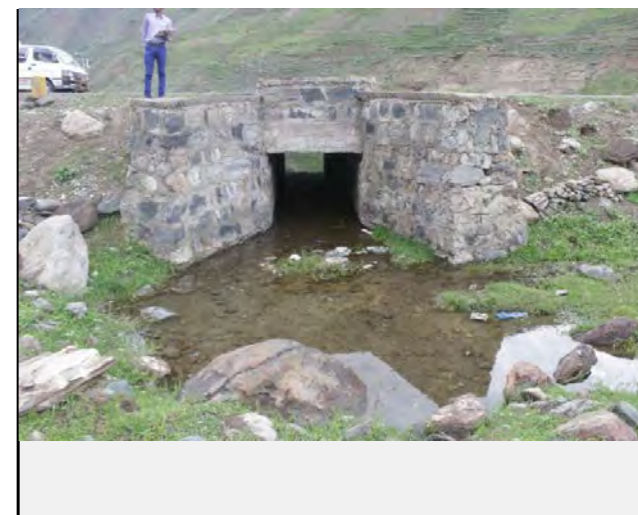
View of Box Culvert at the toe of slope
