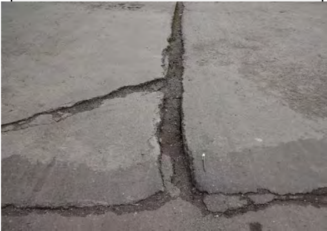
Existing anomalies: Cracks (20cm) was confirmed on the replaced portion of the road.
