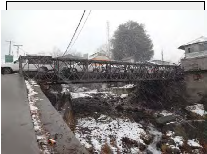
Existing countermeasures: The height of the bridge from the stream bed seems have enough capacity for debris flows at present.
