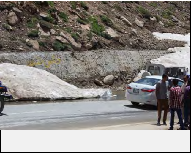
Existing countermeasures / anomalies: Retaining wall has been constructed along the Debris Flow
