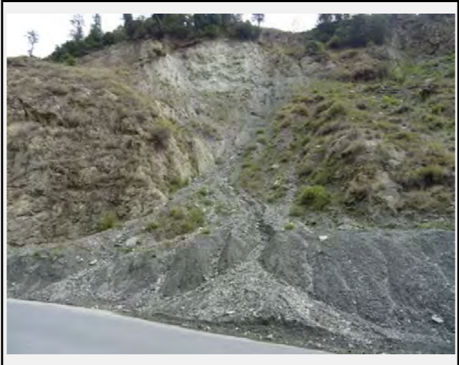
Part of the slope is highly eroded and shows multiple gullies
