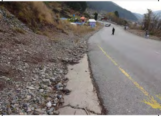
Existing countermeasures: The waterway is filled mostly by the talus.
