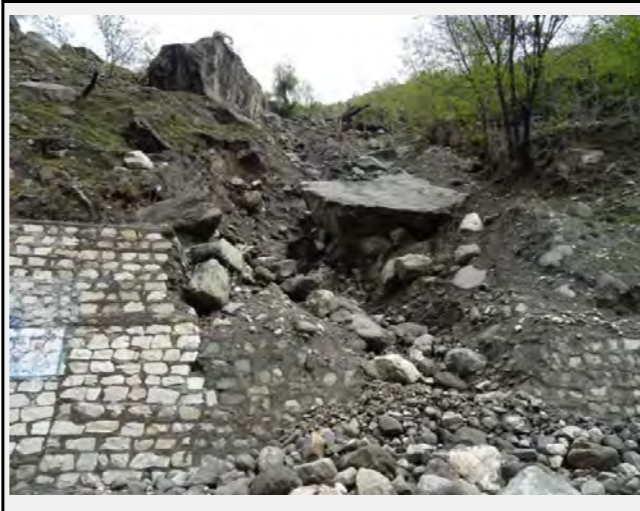
Existing countermeasures / anomalies: The exit of the retaining wall on the mountain side was re-shaped to allow the debris flow. However, this is resulting a steeper angle of the stream. The thickness of the sediment in the stream bed is around 2m
