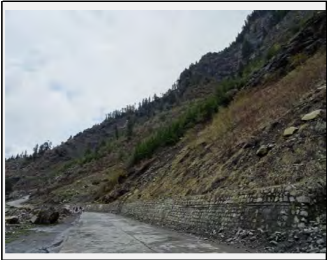
A vertical rock wall of approximately 250 m produces rock falls towards the road. The retaining wall has no effect as a countermeasure for rock falls
