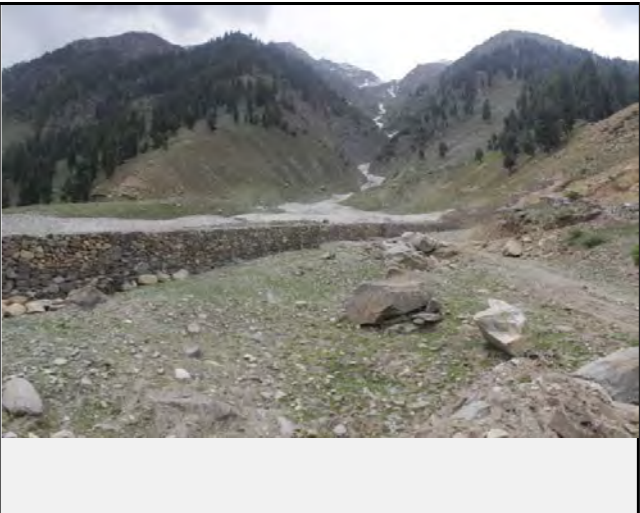
Existing countermeasures / anomalies: Gabion wall has been constructed along the Debris Flow
