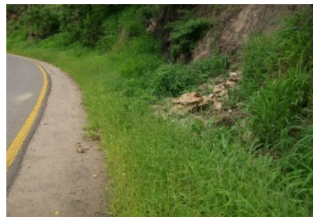
Photo 5.1-7 Gneiss outcrop and fallen rocks along a cut slope (access road on the right-bank side)
