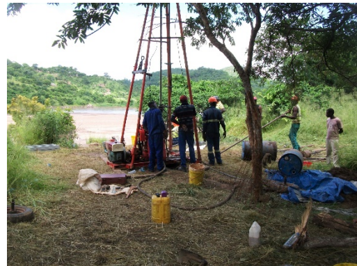
Photo 5.1-11 Boring survey at BH-3 (left bank)
