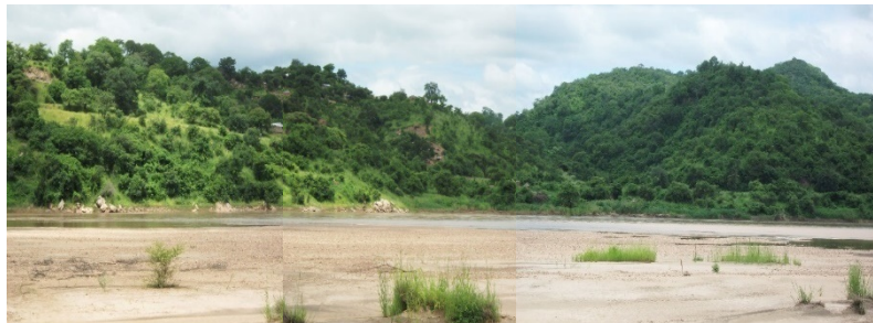
Photo 5.1-3 A distant view of the undercut slope on the right bank side (Lusaka side)
