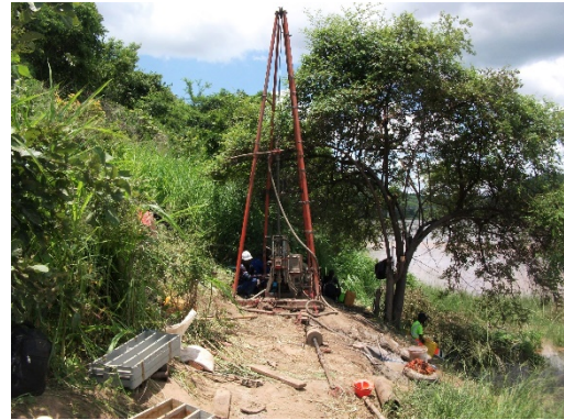
Photo 5.1-9 Boring survey at BH-1' (right bank)
