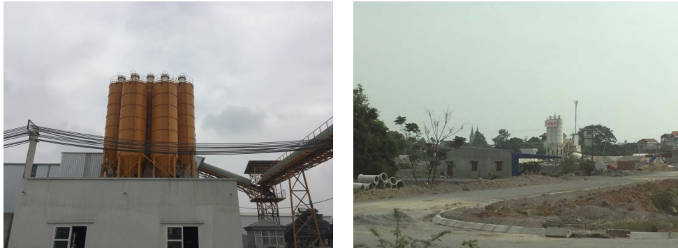
Figure 11.2-2 Photos of Mixed Concrete Plant (1) and (2)
