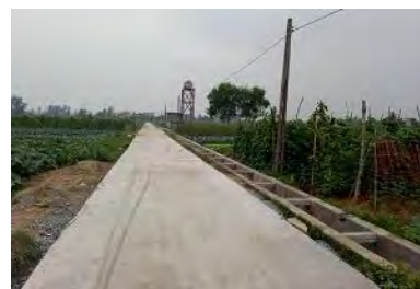
Drainage system built in Village 2 (20th November 2018)
