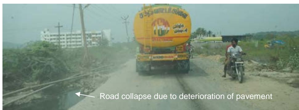
Figure 2.1.17 Problems due to Deterioration of Pavement
