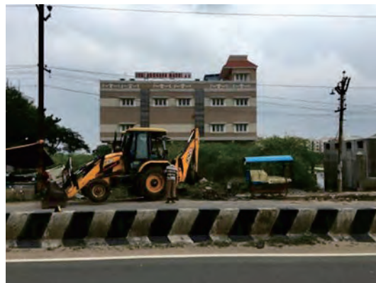
Removal of Sediment from Side Drain
