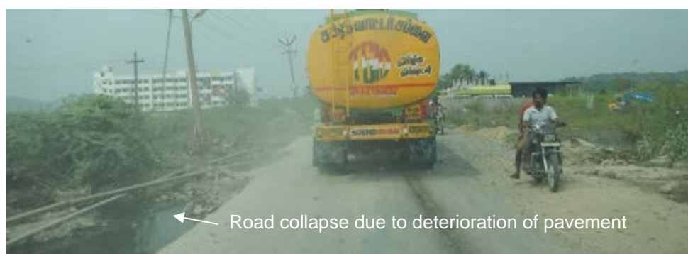
Figure 2.1.17 Problems due to Deterioration of Pavement
