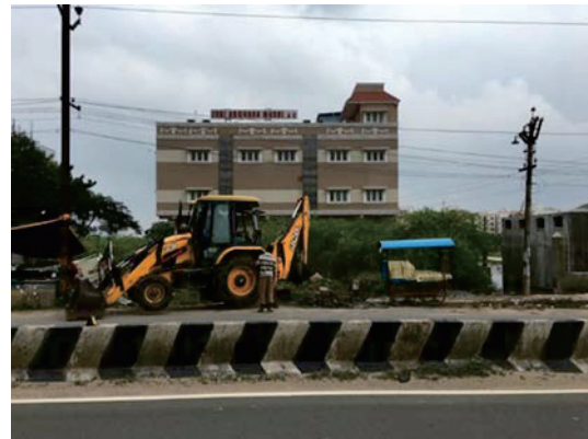
Removal of Sediment from Side Drain
