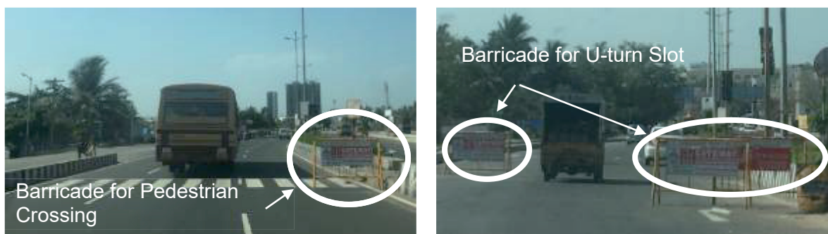
Figure 2.2.3 Installation of Barricades
