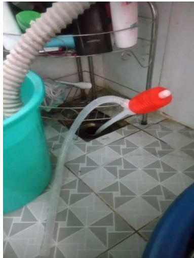
Sampling greywater from bathroom
