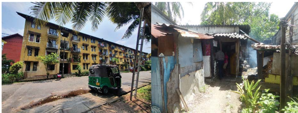
Photo 3: Tsunami housing units in Werasinga
