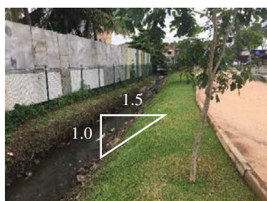
Slope protection with turf and riprap
