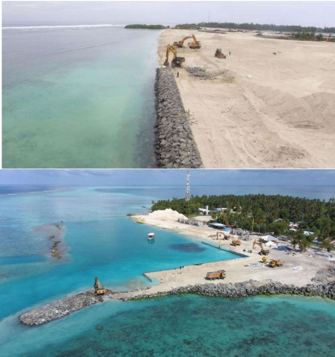
Figure 5.8.32 Installation of the Jetty and Revetment
