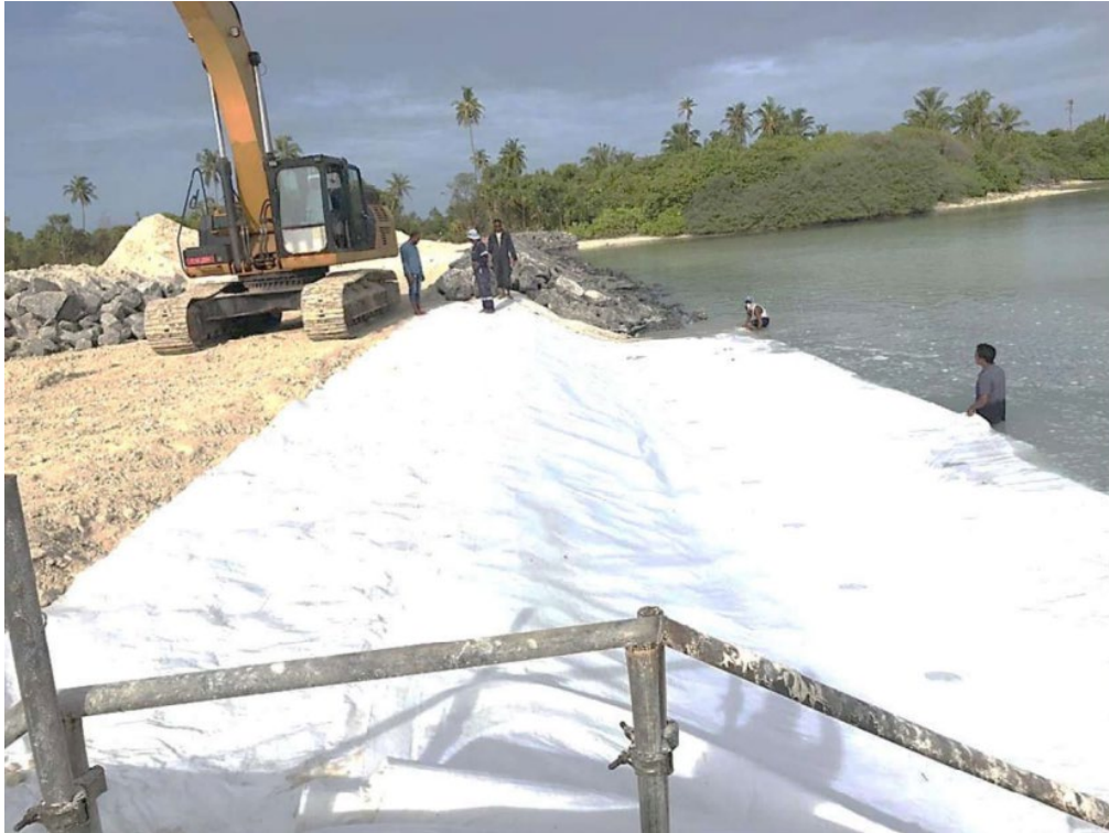
Figure 5.8.36 Installation Situation of Geotextile
