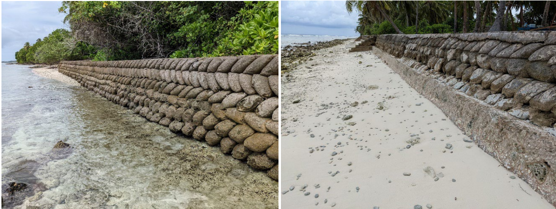
Figure 5.8.33 Installation Situation of the Cement Bag Revetment (left: Gan Island, right: Meedhoo Island)
