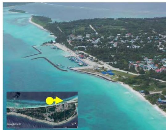
(Erosion on the north side of the fishing port on the lagoon side (north))
