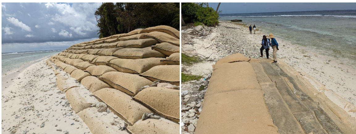
Figure 5.8.34 Installation Situation of the Existing Revetment on Gan Island
