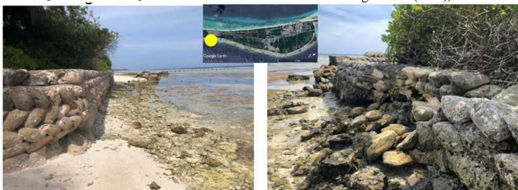
(Beach in front of the Heritage site and collapse of the seawall due to cement bags)
