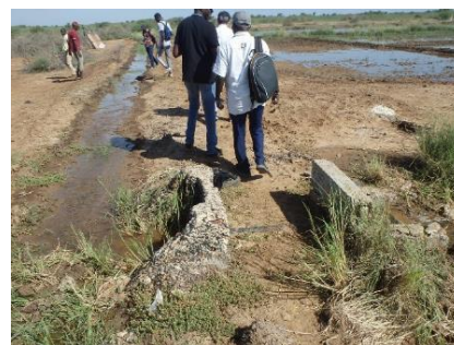
View of secondary canals. Many concreted structures are deteriorating.
