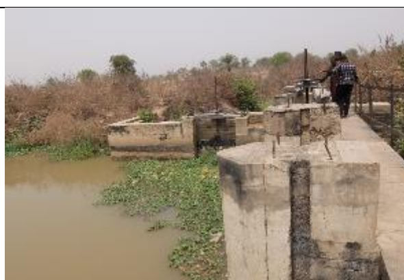
Water intake structure
