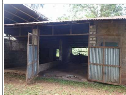
Engineering workshop の外観
