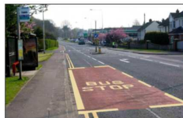
Photo 8f – Typical NI carriageway markings
