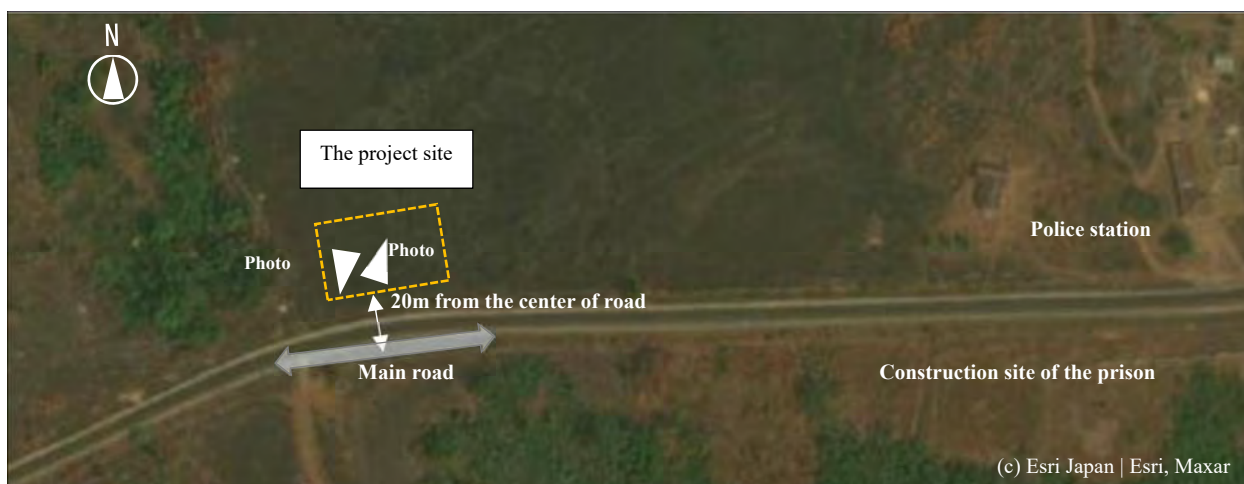
The project site of the York Substation Created from ArcGIS. The project site is a portion of the approximately 8,100 m 2 land that had been reserved in the police station construction plan. The site boundary is 20 m from the center line of the road, taking into consideration the plan to widen the main road.
