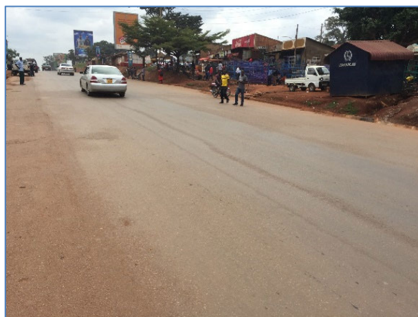
Figure 4-4 Faded out Road Markings and Lack of Road Marking
