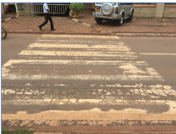
Figure 4-4 Faded out Road Markings and Lack of Road Marking
