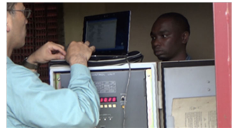
Photograph 4-4 An OJT Scene of Re-configuration of Signal Timing
