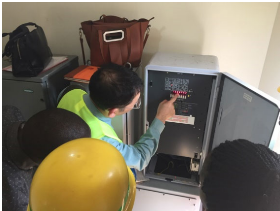
Photograph 6-1 Modifying of the Signal Timings Using Control Panel
