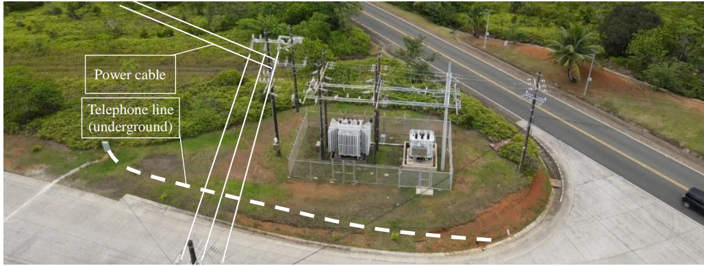
Panoramic view of the existing Kokusai substation and the construction site
