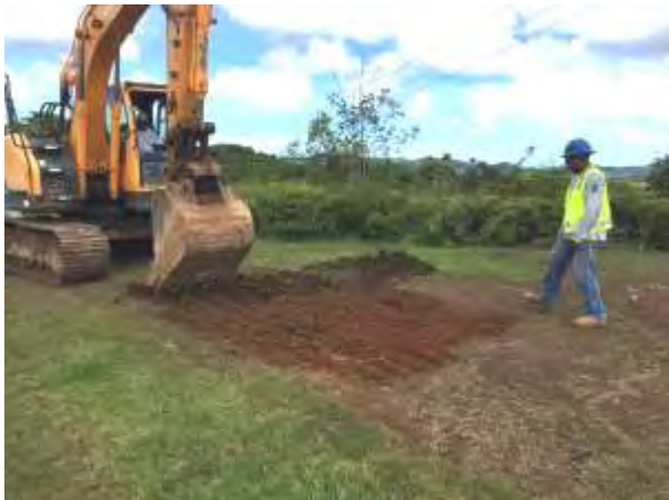
Digging of Test Pit
