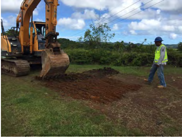
Digging of Test Pit
