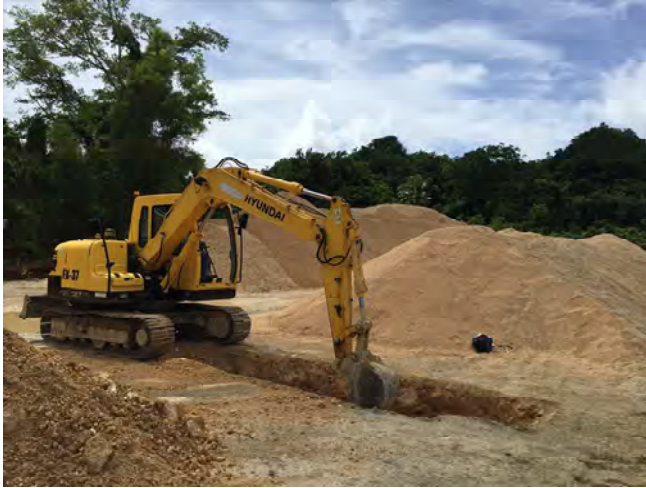
Digging Test Pit
