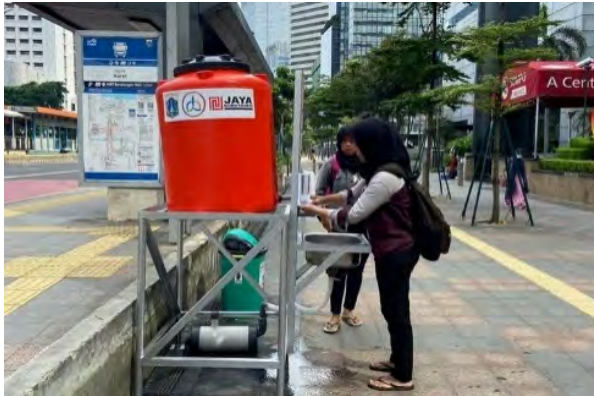
Figure 5.1.14 Water Tank for Handwash along Sidewalk
