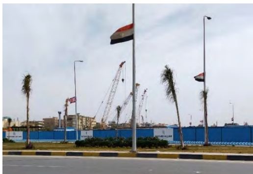
Metro station under construction adjacent to the Pyramids (February 2022)
