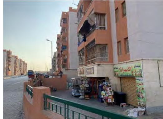
One of the few shops in Asmarat. The district has almost no workplaces and people are unemployed or work in the surrounding area or in the city center, but transportation is limited. (October 2021)
