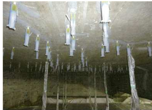
(Bottom Surface of RCC Slab)
