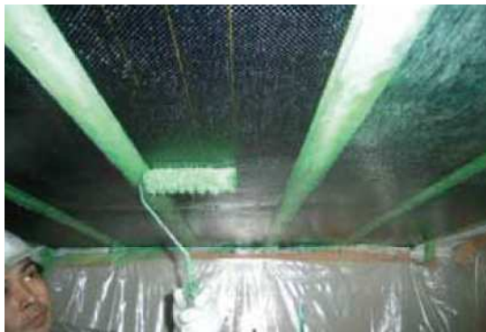
(Adhering CFRP Sheet)
