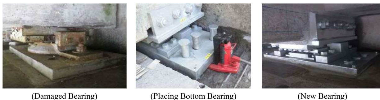
Figure 5.86 Example of Construction of Replacement of Bearings (PSC Girder)
