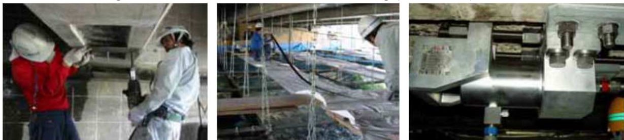
(Drilling Anchoring Holes)
