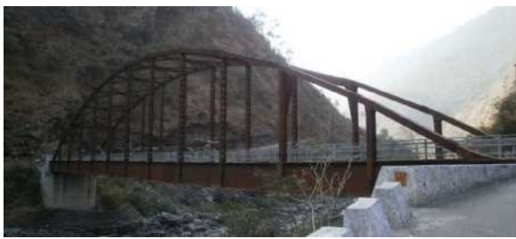
Steel Langer Arch Bridge (Wakleytar in Wangdue)
