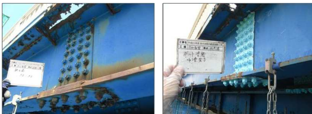
(before Replacing Bolts) (After Replacing Bolts with Repainting Splice Plate)
