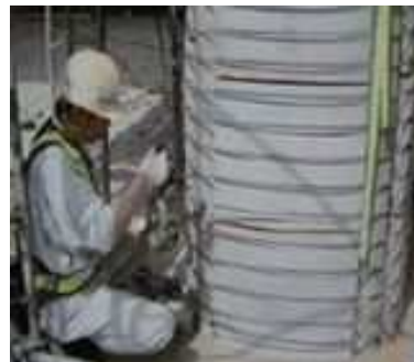
(Load Tension to Spiral Tendon)
