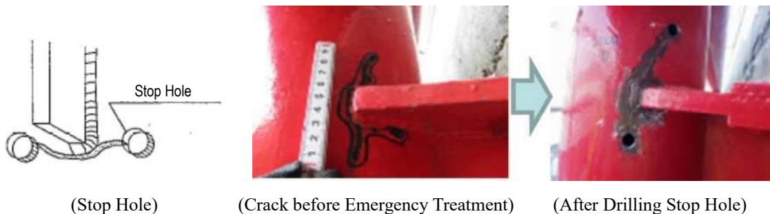
Figure 5.74 Example of Construction of Stop Hole
