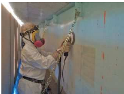
(Scraping the existing Paint)
