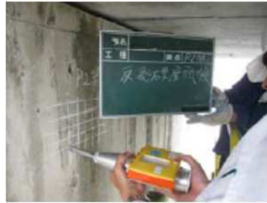
Figure 5.12 Example of Rebound Hardness Test by Schmitt Hammer
