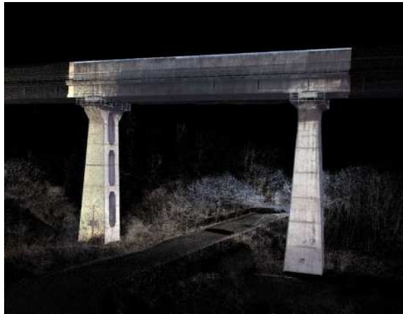
Figure 5.3 Example of Collected Data of Mobile 3D Laser Scanner
