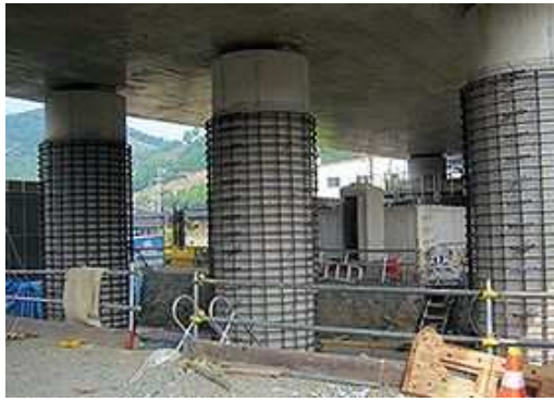
(Rebar Arrangement)
