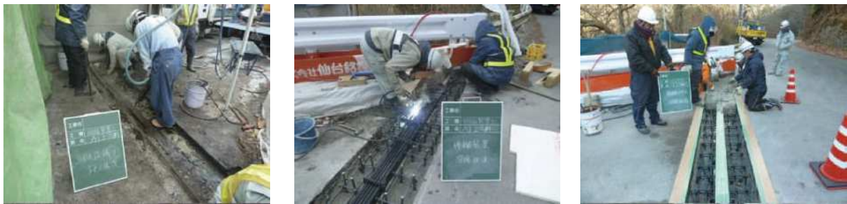
(Removing) (Anchor Bar, Rebar Arrangement) (Casting Rapid Hardening Concrete)
