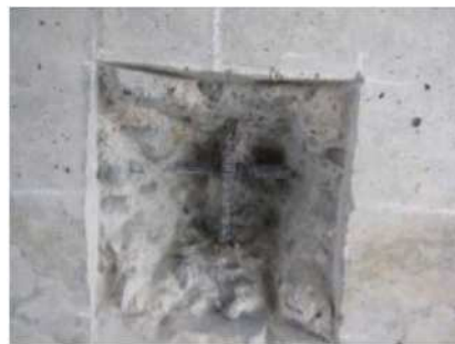
Figure 5.17 Example of Direct Observation by Chipping Cover
