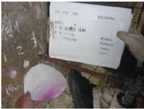
(Drilling a small holes)
