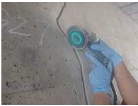
(Cutting the Ditch with Electric Cutter)
