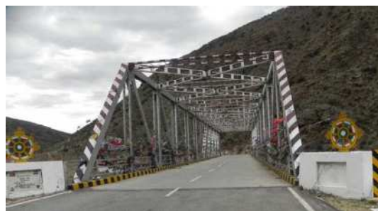
Steel Truss Bridge (Isuna in Paro)
