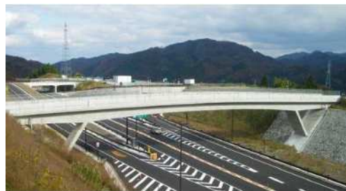
Rigid Frame Bridge
