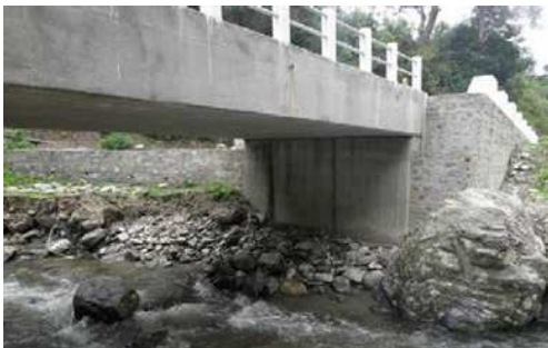
Slab Bridge (NgashayZam in Wangdue)
