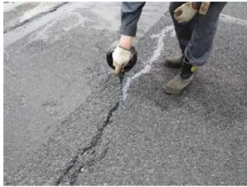
Figure 4.9 Example of Crack Patching of Wearing Course
