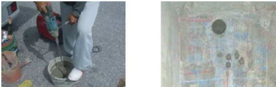
Figure 5.10 Examples of Refilling the Hole after Collecting the Core Sample
