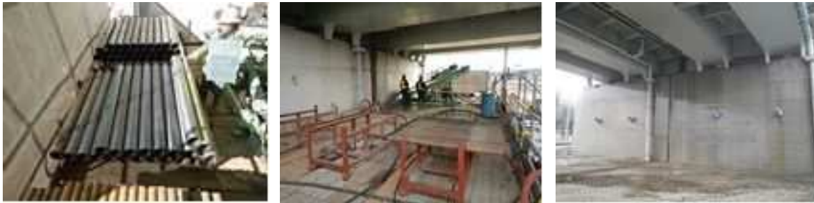
(Casing of Ground Anchor)
