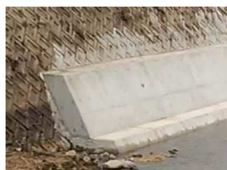
(RCC Retaining Wall)
