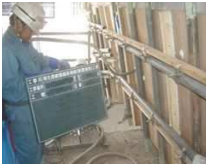
(Grouting Non-shrinkage Mortar)
