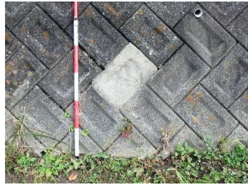
(Re-patching of Masonry Structure)
