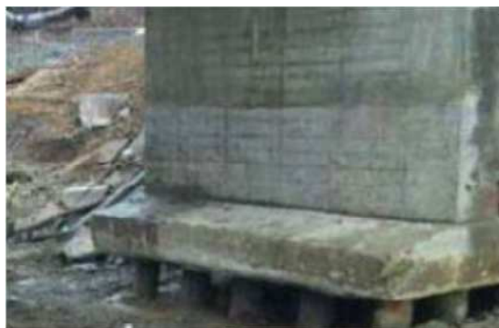
Figure 5.6 Example of Scouring which requires Detailed Observation
