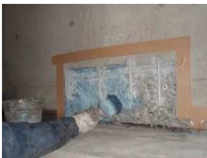
(Rustproofing of Rebar, Primer Coating)
