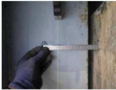
(Measuring Inclination by Plumb-bob and Steel Ruler)
