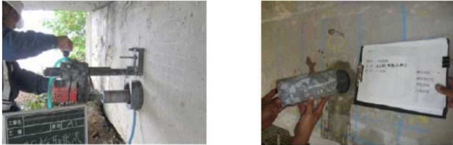
Figure 5.9 Examples of Collecting Core Sample from Substructure
