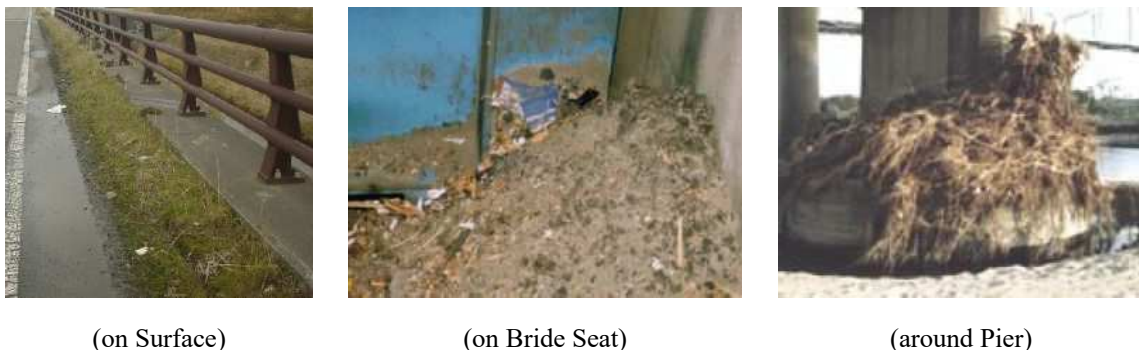
Figure 4.5 Example of Sediment Deposition
