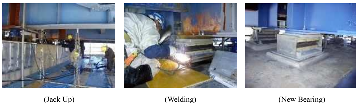
Figure 5.85 Example of Construction of Replacement of Bearings (Steel Plate Girder)
