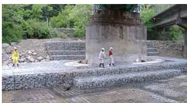
(Riverbed Protection by Gabion)
