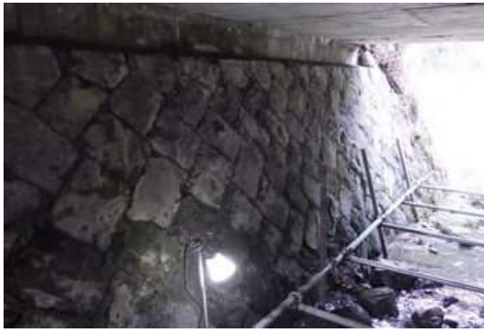
(Repair of Cracks in front of Abutment)
