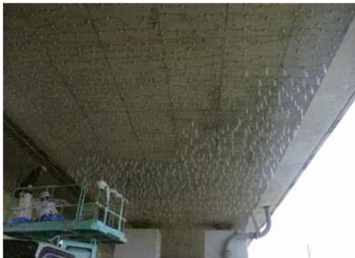
(Bottom Surface of Voided Slab)
