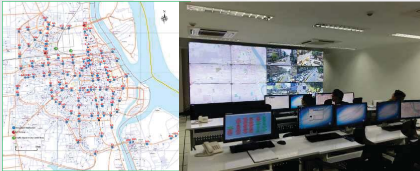
Traffic Management System in Phnom Penh funded by JICA
