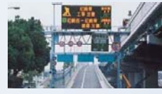
Variable Message Signboard at on-ramp
