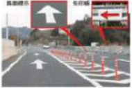
Large arrow road markings, rubber poles, high-intensity arrow boards (highway main line confluence)
