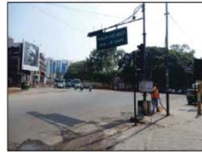
Absence of Traffic Lane and Other Indications in Intersection
