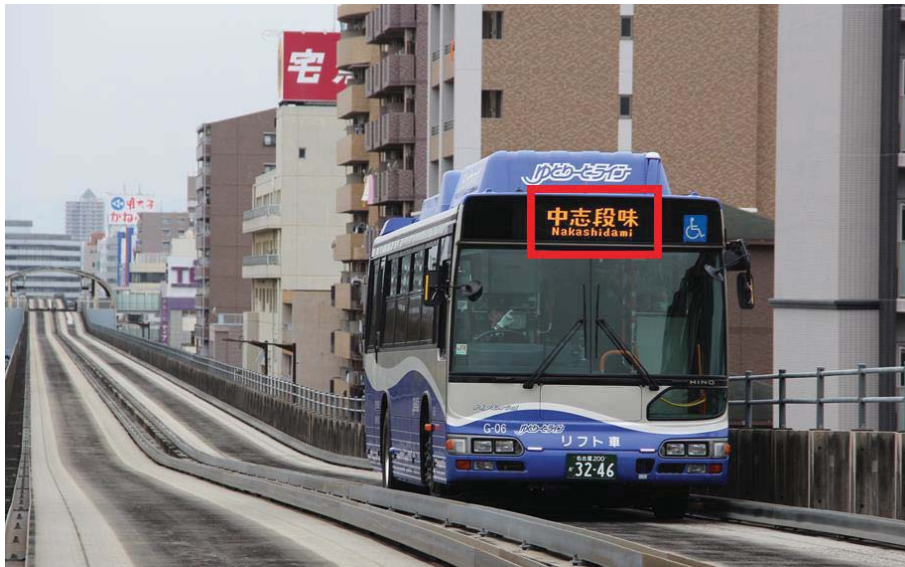
BRT Lines in Nagoya and information of next station and line written
