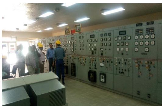
Site visit to Kotri TPS (3)
