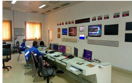
Site visit to Nandipur TPS (3)
