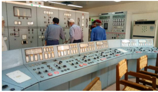
Site visit to Faisalabad TPS (3)
