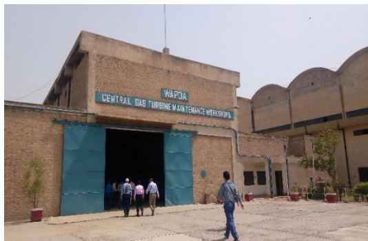
Site visit to Central Gas Turbine Maintenance Workshop (1)
