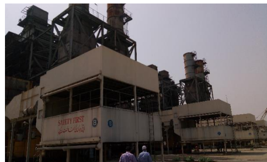
Site visit to Faisalabad TPS (2)
