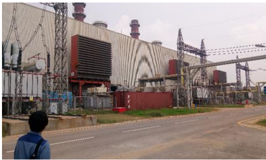
Site visit to Nandipur TPS (2)
