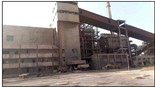
Site visit to Lakhra TPS (2)
