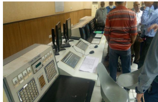
Site visit to Kotri TPS (2)
