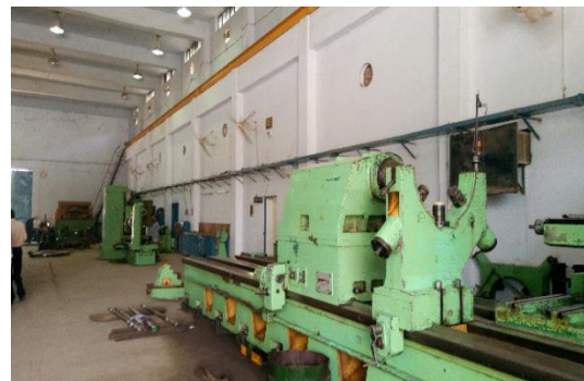
Site visit to Central Gas Turbine Maintenance Workshop (2)
