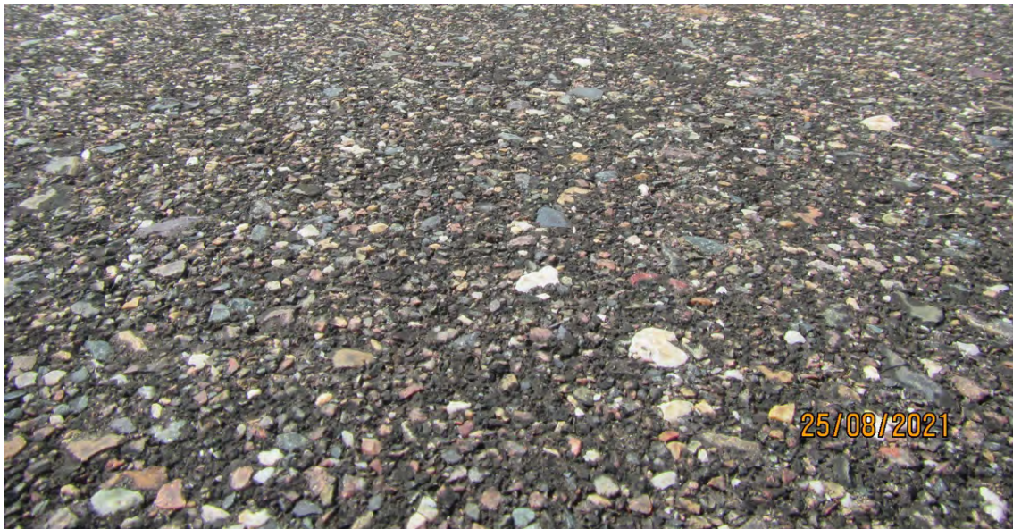
Figure 4.21 Pavement Surface Condition of Taxiways
