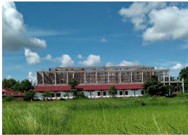
Temple annex (under construction)
