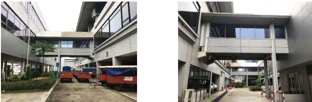
Figure 5.2 Space between the Departure Concourse and the Main Building
