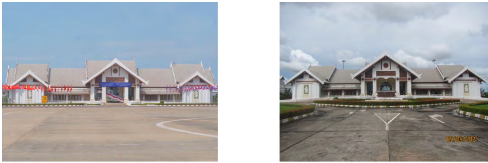
Figure 2.77 VVIP Terminal (left: from Airside, right: from landside)
