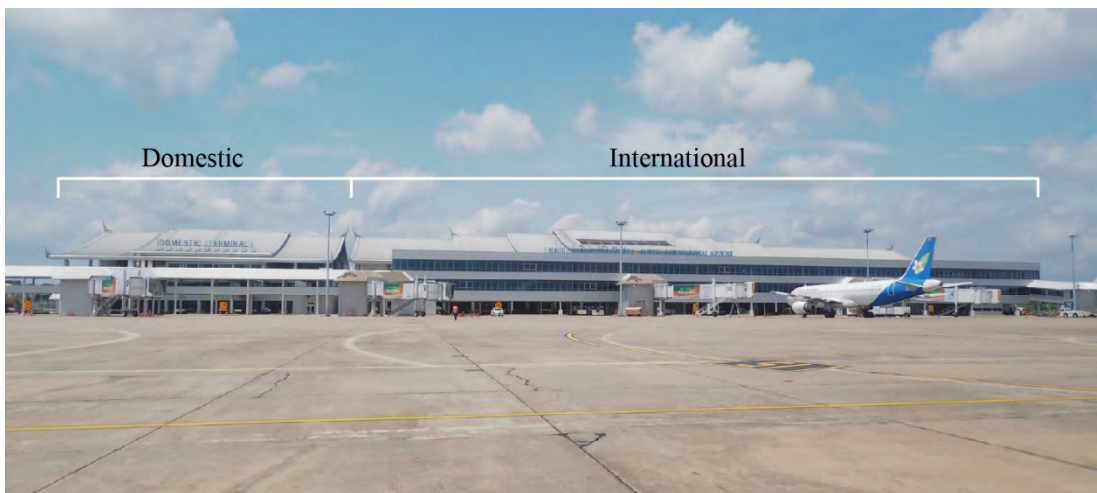
Figure 2.51 International and Domestic Passenger Terminal Building from Airside
