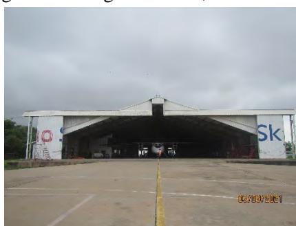
Figure 2.84 Lao Skyway Hangar
