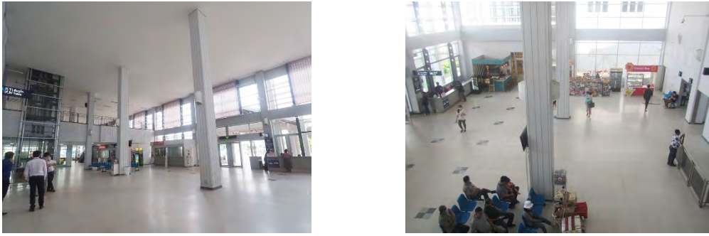
Figure 2.76 Arrival Lobby in DPTB
