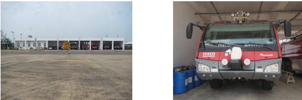
Figure 2.85 Fire-Fighting Station (left) and Fire-Fighting Vehicles (right)
