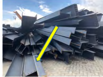
Need to prevent collapse
