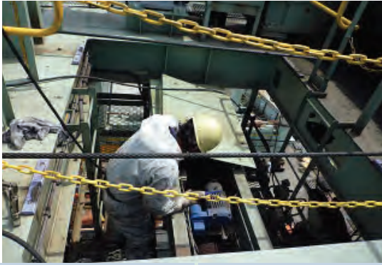
Pad of Disc brake and other parts of Main Hoist Brake are cleaned by air-brush.
