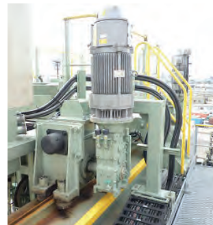
Clearance between Traverse Guide Rollers and Trolley Rail is checked.
