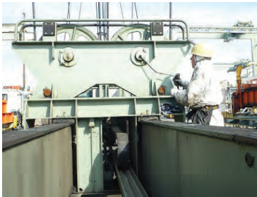
Refueling of grease to Sheave bearing
