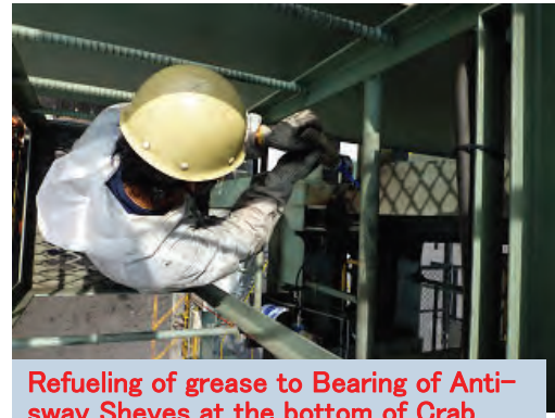
Refueling of grease to Sheave bearings for Anti-sway and Main Hoist
