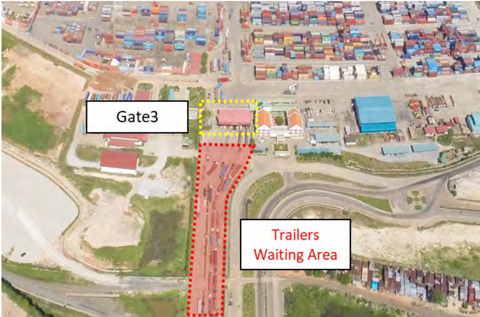
Picture 1.2-6 Gate3 and trailers waiting area
