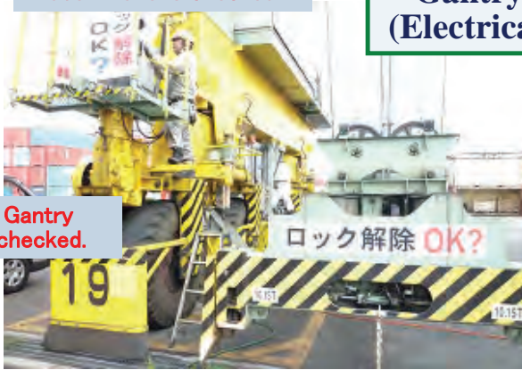
Clearance of pad of Travel Brake is checked.
