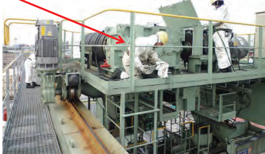
Refueling of grease to Bearings of Main Hoist and Anti-sway Sheaves
