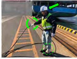
Safe wire works
