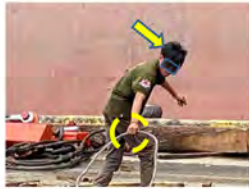
No safety equipment
