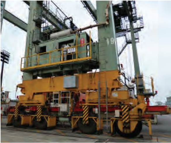
Gantry Travel Part (D-G Set Side)
