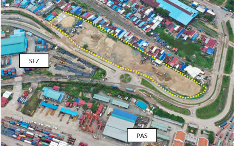
Picture 1.2-3 Parking yard near Gate 3
