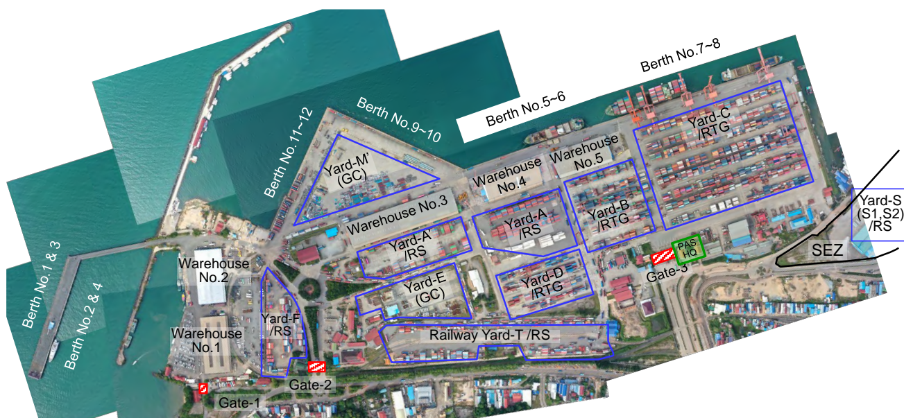
Figure 2-2 Major Facilities of the Sihanoukville Port (December 2021)
