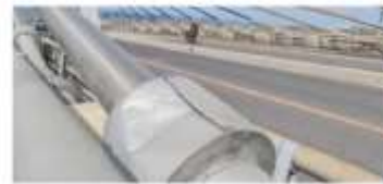
DEFORMED DAMPER DRUM
