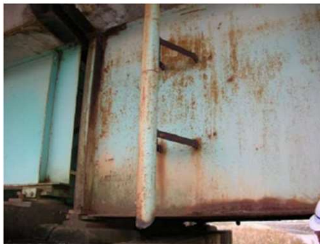
Figure 7.15 Example of Girder End Corrosion Due to Water Leakage from an Expansion Device 89
