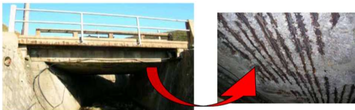
Figure 7.16 Examples of Salt Damage 90
