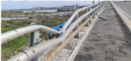
Damaged Railings and Post
