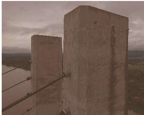
Figure 11.25 Disconnection of Cable Cover at the Main Tower
