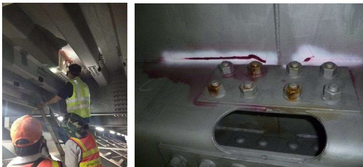
Figure 11.44 Cracks in steel slab and U-rib reinforcement
