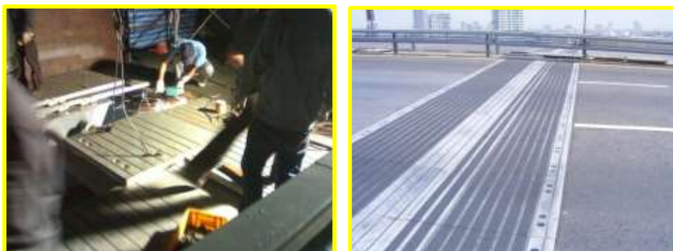
Figure 11.39 Replacement of an Expansion joint (2010)
