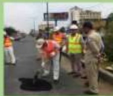
Repair of potholes using Excel Patch
