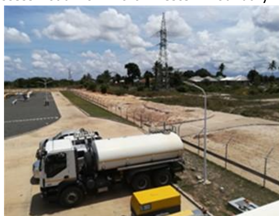
Figure 12.4-10 Kinyerezi energy complex: Southern boundary
