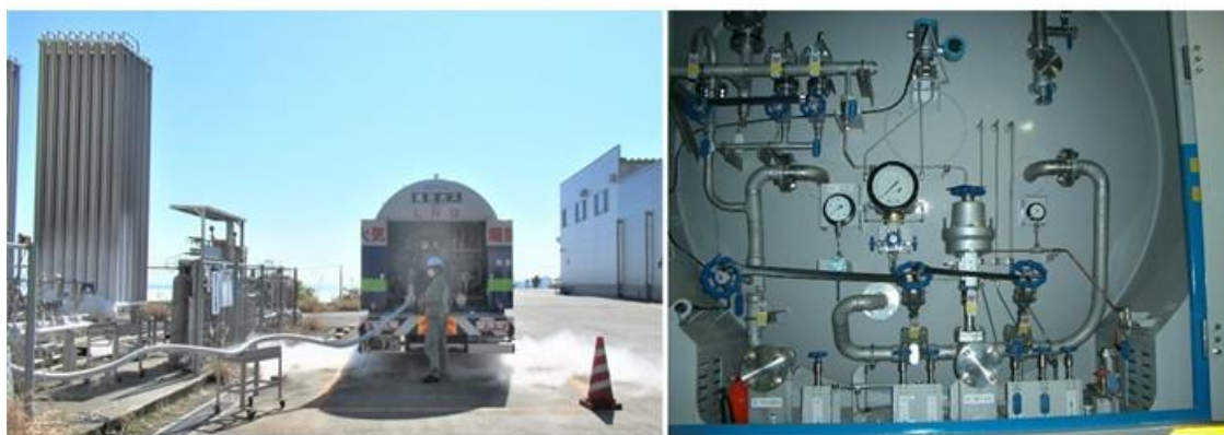
Figure 10.3-3 Valves and Gauges of LNG Tank-truck/container
