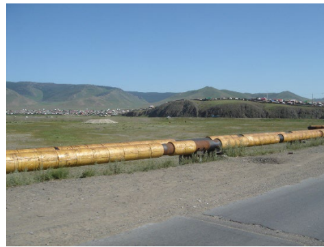
Overhead Pipes Undergoing Insulation Repairs
