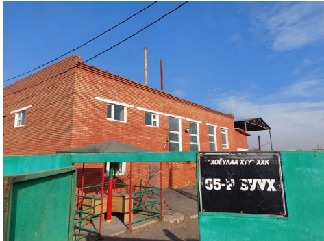
Heat Supply Facilities
