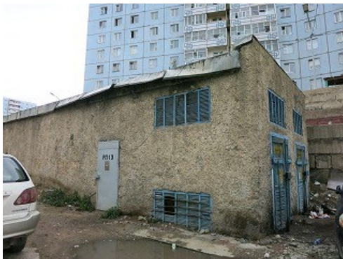
Exterior of Switching Station
