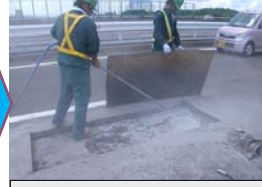
Clean up the surface with blower
