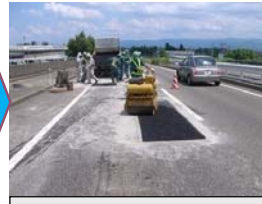
Compaction with hand roller (1t)
