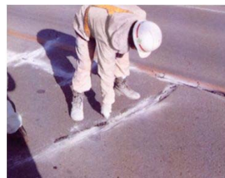
Fill up fine aggregate
