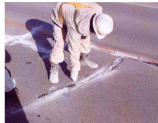
Fill up fine aggregate
