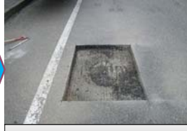
Remove the damaged area
