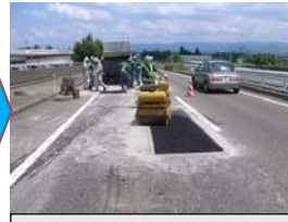
Compaction with hand roller (1t)
