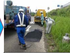
Spreading asphalt mixture
