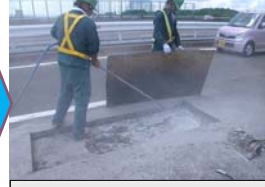
Clean up the surface with blower
