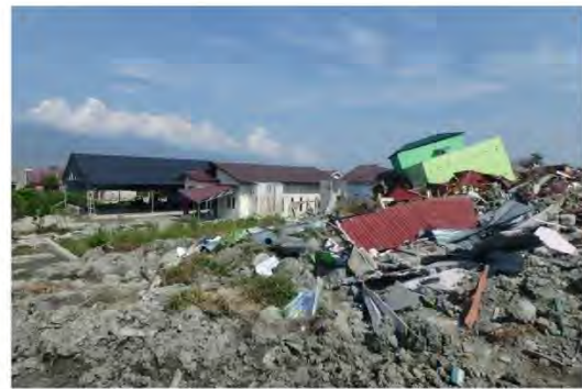
Fig. 16. House and buildings outside the flow area are undamaged (Petobo).
