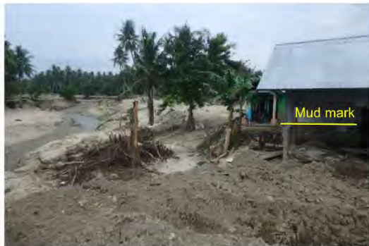
Fig. 23. Mud mark on the house indicates the likely thickness of the mudflow (Jono Oge).
