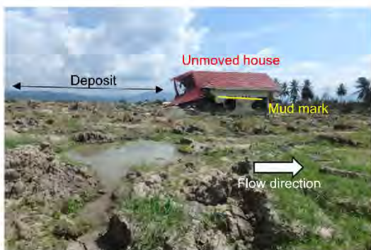
Fig. 26. Thick sediment on the upstream side of the unmoved house in Jono Oge.
