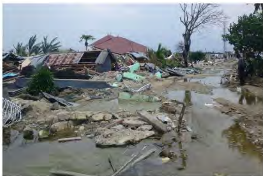
Fig. 9. Water inundation appeared after the earthquake (Balaroa).
