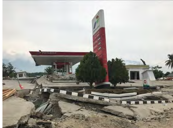
Building Affected by Liquefaction in Lolu, Sigi
