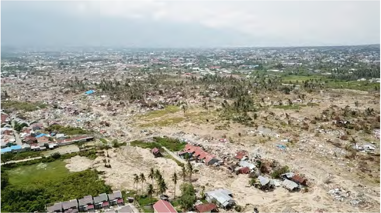
Petobo Landslide-affected Area (Aerial view by drone)
