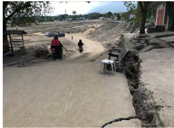
Landslide-affected area Balaroa, Palu
