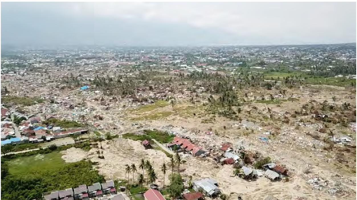
Petobo Landslide-affected Area (Aerial view by drone)
