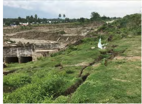
Upper part of of Liquefaction Landslide in Sibalaya, Sigi
