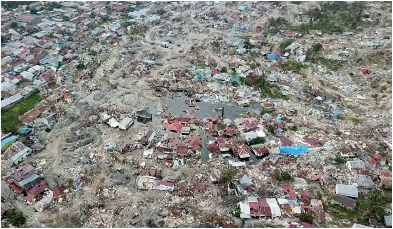
Balaroa Landslide-affected Area (Aerial view by drone)
