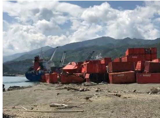
Container Port near Lampowau (West Coast)
