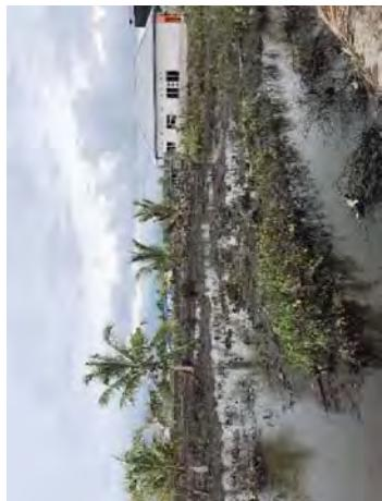
In this coastal area near the epicenter of September 28, 2020, the ground has subsided. Since subsidence of more than 2 m has occurred, flood damage due to storm surge and drainage failure has occurred. Inundation occurs every day for several days before and after the spring tide, causing inundation of houses and disruption of national roads.
