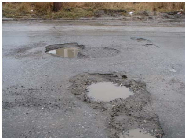
Figure I-5-1-4 Shape of Potholes
