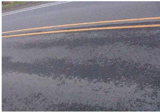
Figure I-5-1-5 Shape of Bleeding
