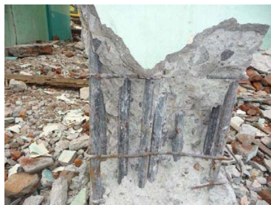
Fig-89: Lap at Bottom of Column
