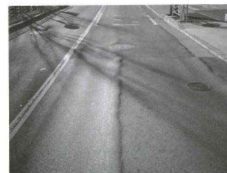
Figure I-5-1-3 Photographic Examples of estimated levels of rut depths by Visual Inspection
