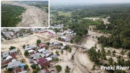
Fluidized sediments generated by liquefaction-landslide flowed into the river, and sediment flooding has occurred.
