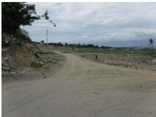
Liquefaction in Balaroa
