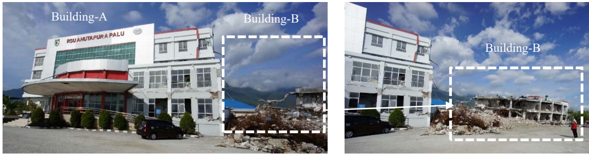
Figure 3-37 Building-B which slid away and totally collapsed
