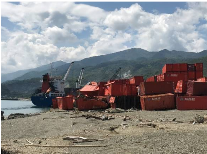
Damaged Port Facilities in the Palu Bay (The Photo is SAMAS Container Jetty on the Left Shore of Palu Bay)
