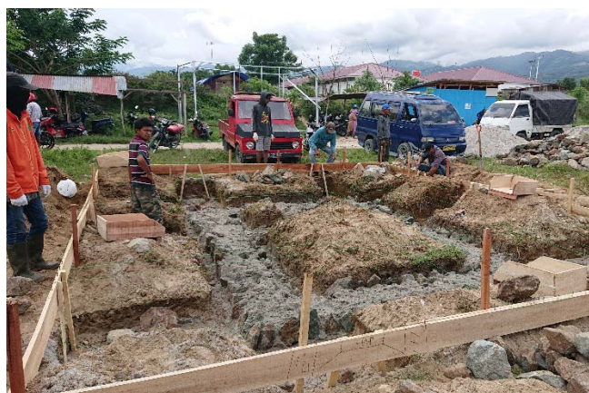
Pilot Project Activities in M'panau Village (Output 4)
