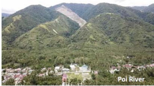
Large-scale Landslide (mountain collapse) has occurred. There is a high risk of sediment disaster caused by earthquakes and heavy rainfall.
