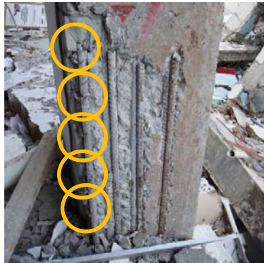
Figure 3-41 No Hoop Bar for Column
