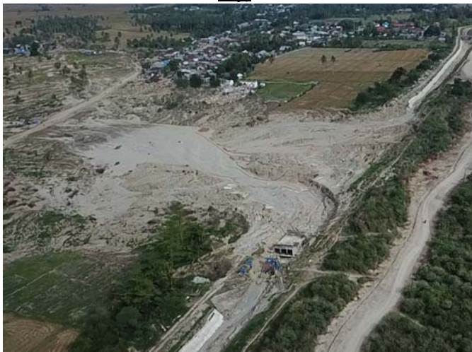
Damaged in Sibalaya Area by Nalodo (Sigi Regency, Drone Shooting)
