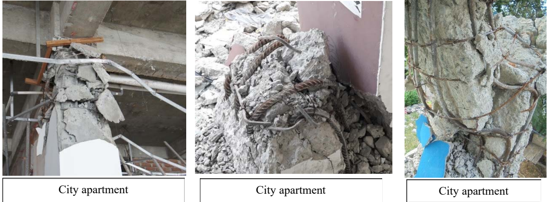
Figure 3-44 Poor Quality Concrete
