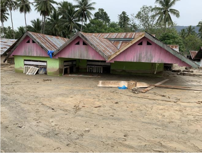
Damaged Caused by Floods and Landslides (Bangga River, Sigi Regency)
