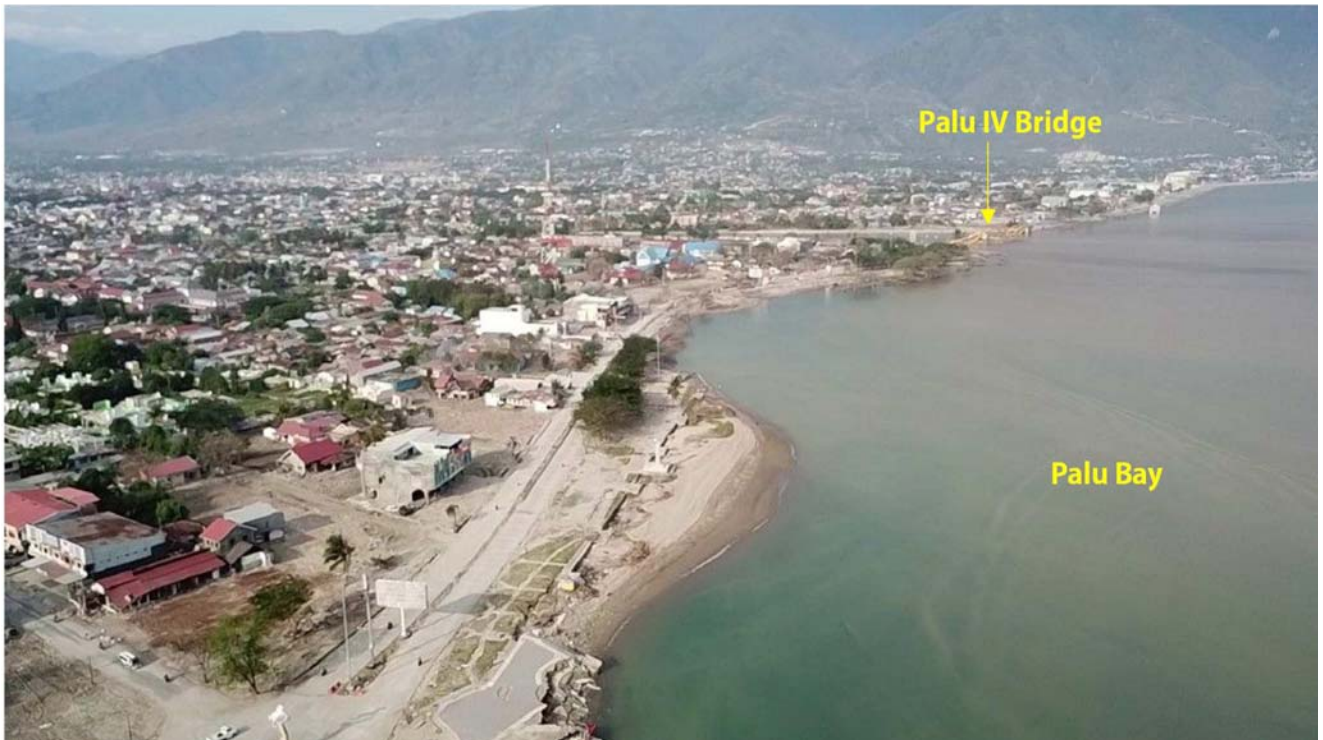
Condition of the Coastal Area of Palu Bay After the Disaster (Right Shore Side, Drone Shooting)
