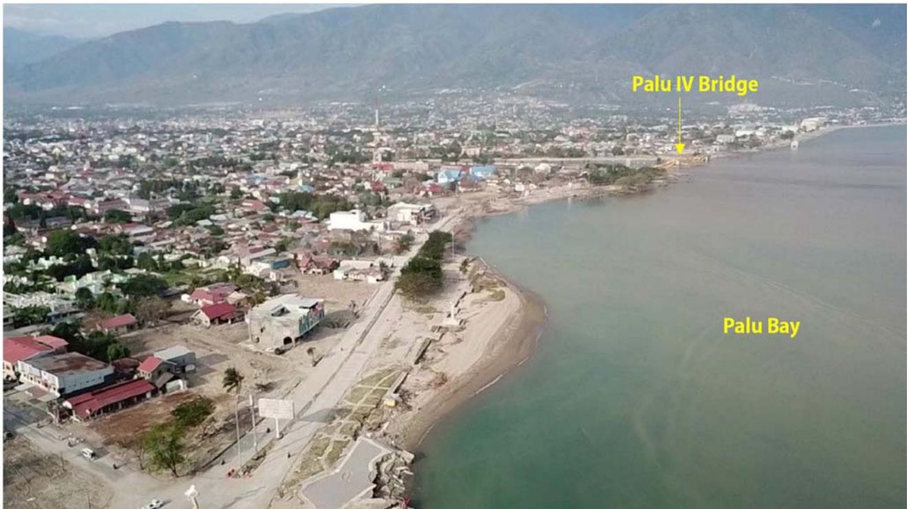
Condition of the Coastal Area of Palu Bay After the Disaster (Right Shore Side, Drone Shooting)
