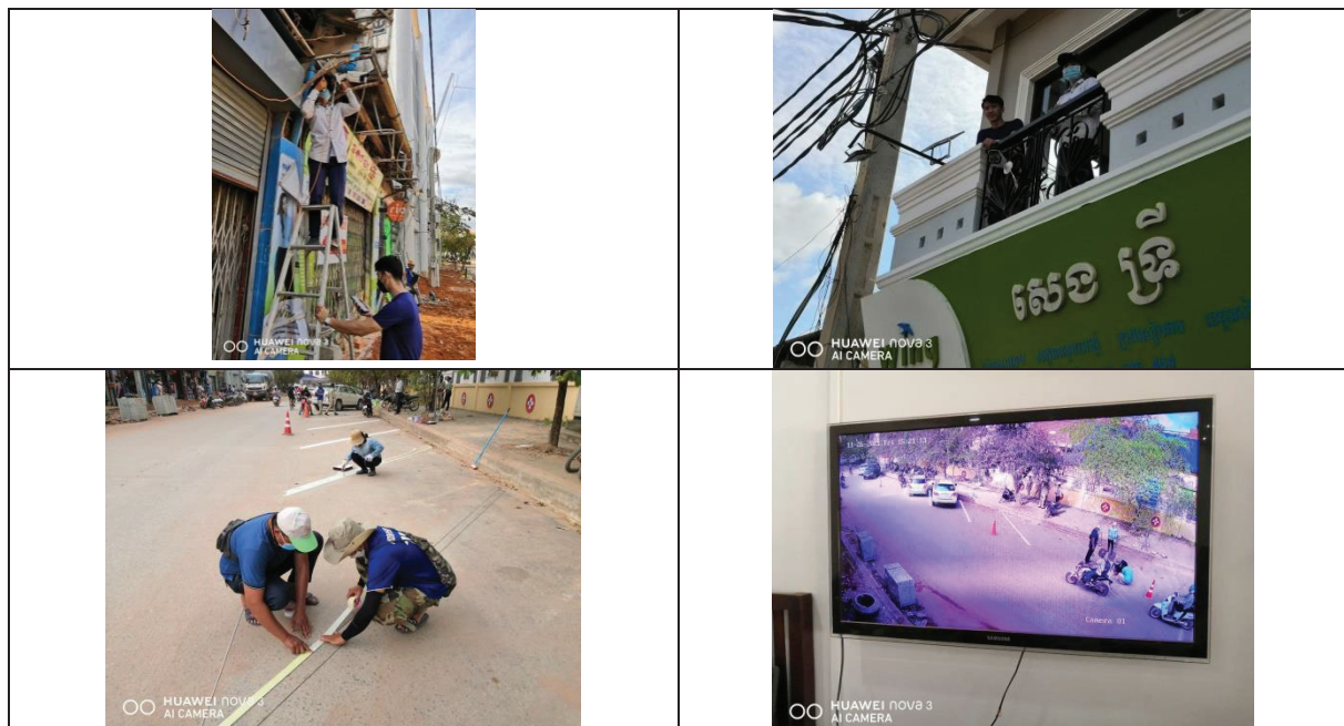
Figure 1-3 Installation Work of Equipment and Parking lot marking
